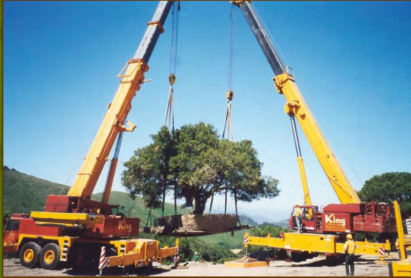
Giant Coast Live Oak Relocated via Dual Crane Lift
