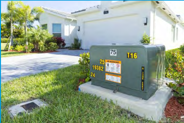
Pad-mounted transformer
