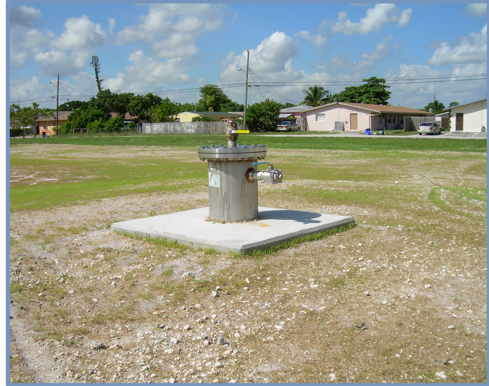
Floridan Aquifer Test Wells (City Constructed Two Wells)
