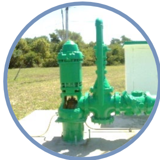
Water Supply Testing
