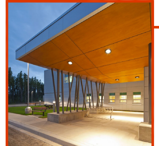
WOOD PANEL SOFFIT ACCENTS
