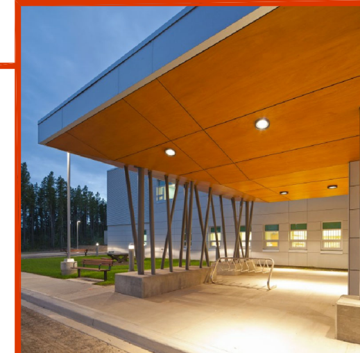
WOOD PANEL SOFFIT ACCENTS
