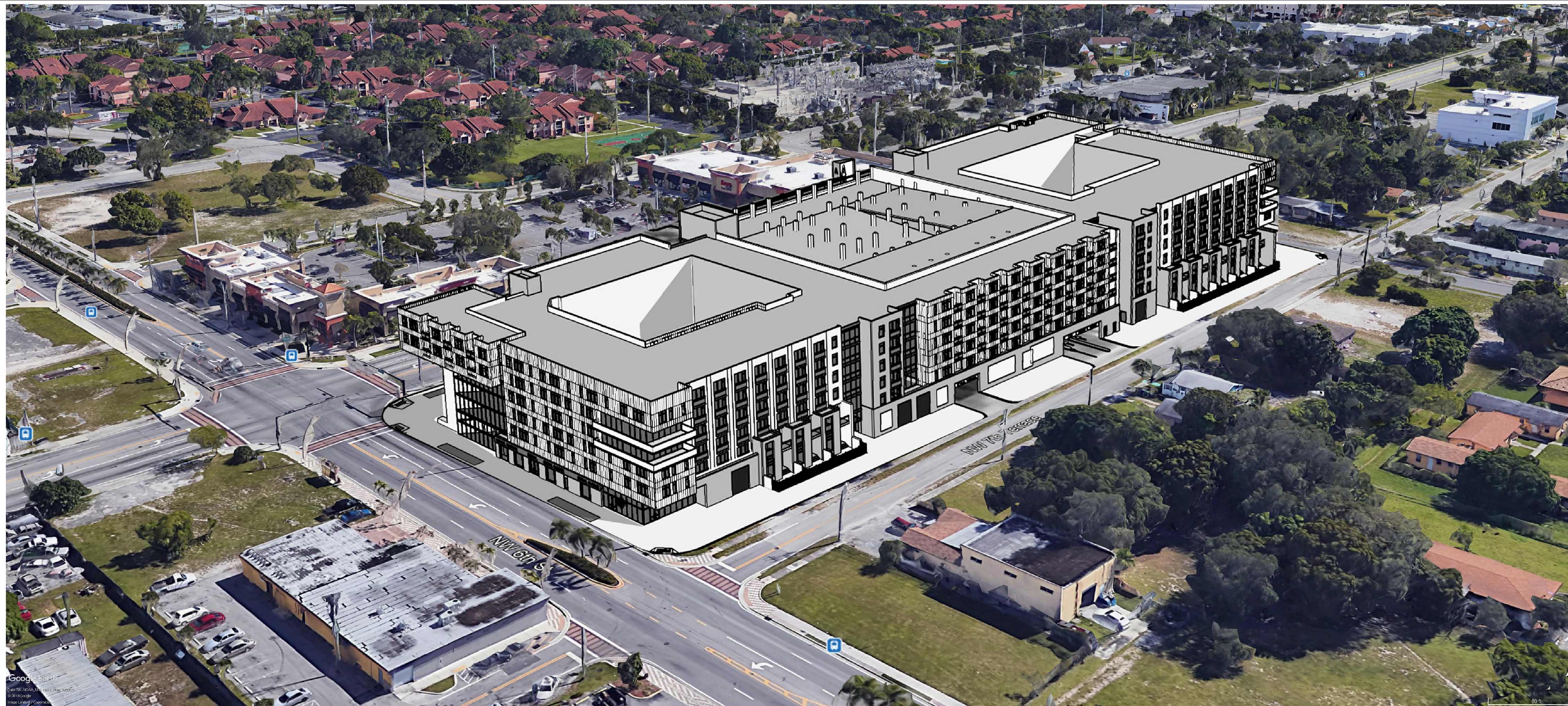
VIEW LOOKING SOUTH EAST
