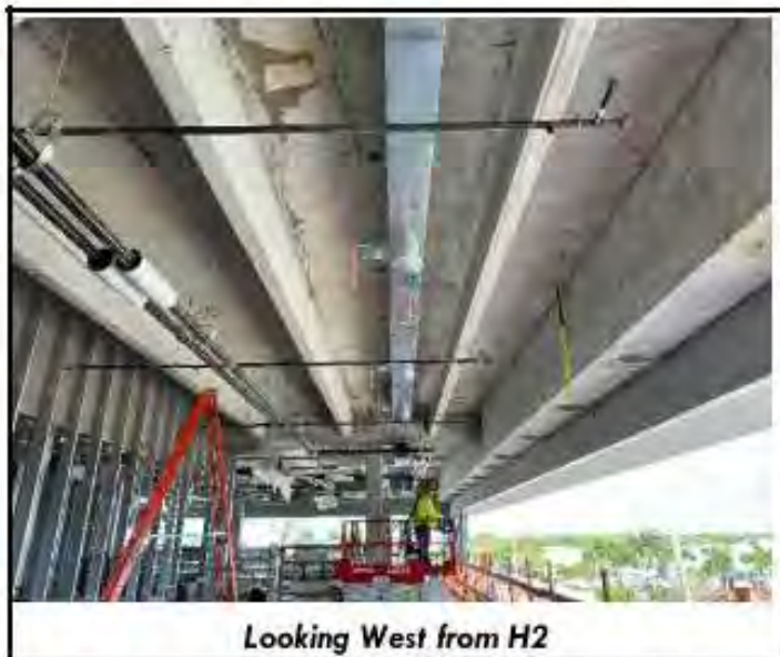
Figure 32. Photograph from Threshold Inspection Report No. 127 showing underside of roof slab at north end of the building showing water which has filtered through from the top of the roof slab at cracked slab locations.
