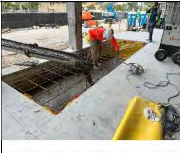
Figure 50. Photograph from Threshold Inspection Report No. 142 showing concrete placement at column footing enlargement.
