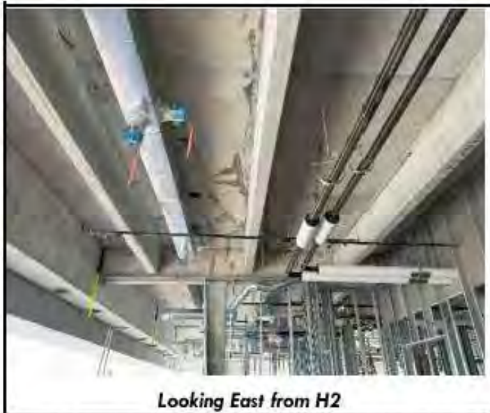
Figure 31. Photograph from Threshold Inspection Report No. 127 showing underside of roof slab at north end of the building showing water which has filtered through from the top of the roof slab at cracked slab locations.
