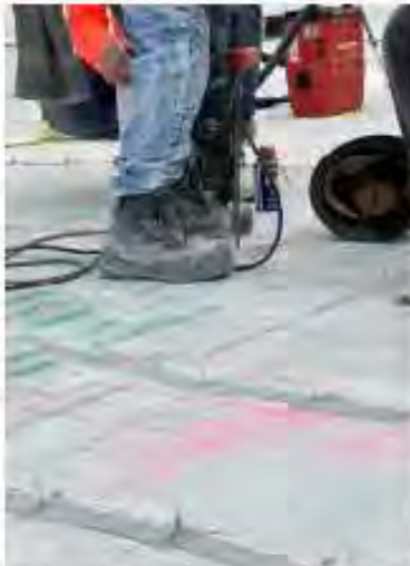
Figure 54. Photograph from Threshold Inspection Report No. 201 showing epoxy crack injection of cracks in roof slab.
