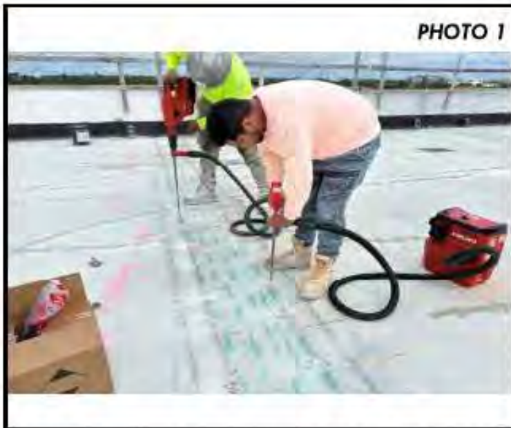
Figure 51. Photograph from Threshold Inspection Report No. 200 showing drilling of holes for inverted "U" shaped stirrups in upturned beams.
