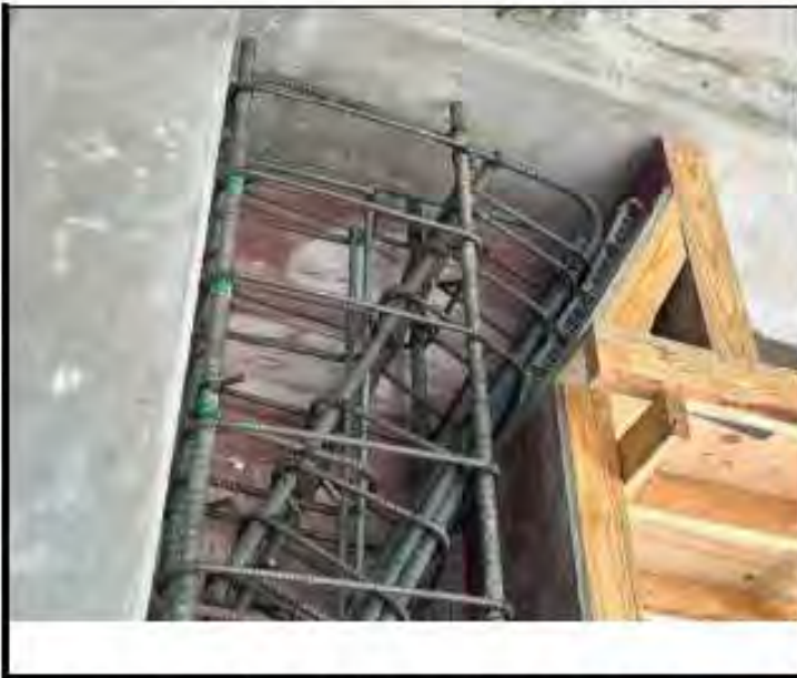
Figure 42. Photograph from Threshold Inspection Report No. 140 showing completed reinforcement installation at third story column enlargement.
