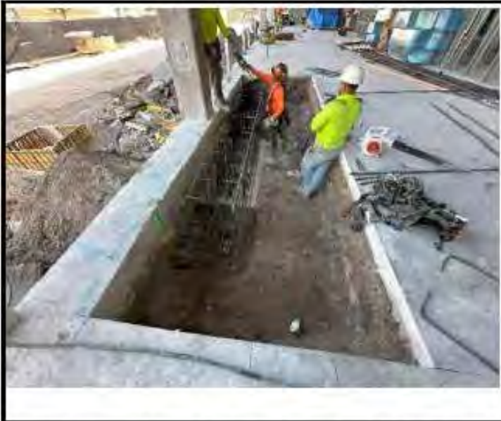
Figure 43. Photograph from Threshold Inspection Report No. 140 showing continuing work on column footing enlargement.
