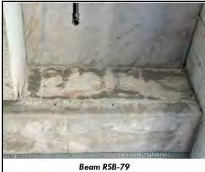
Figure 28. Photograph from Threshold Inspection Report No. 125 showing conditions at underside of roof slab and at beam RSB-79 (gridline J-2) at north end of building.
