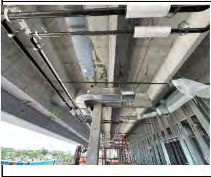
Figure 33. Photograph from Threshold Inspection Report No. 127 showing underside of roof slab at north end of the building showing water which has filtered through from the top of the roof slab at cracked slab locations.
