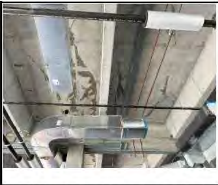
Figure 34. Photograph from Threshold Inspection Report No. 127 showing underside of roof slab at north end of the building showing water which has filtered through from the top of the roof slab at cracked slab locations.
