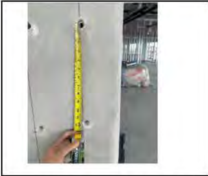
Figure 35. Photograph from Threshold Inspection Report No. 137 showing holes drilled in the north side of column H-2 to receive rebar dowels as part of the rectification of the column and roof structure.
