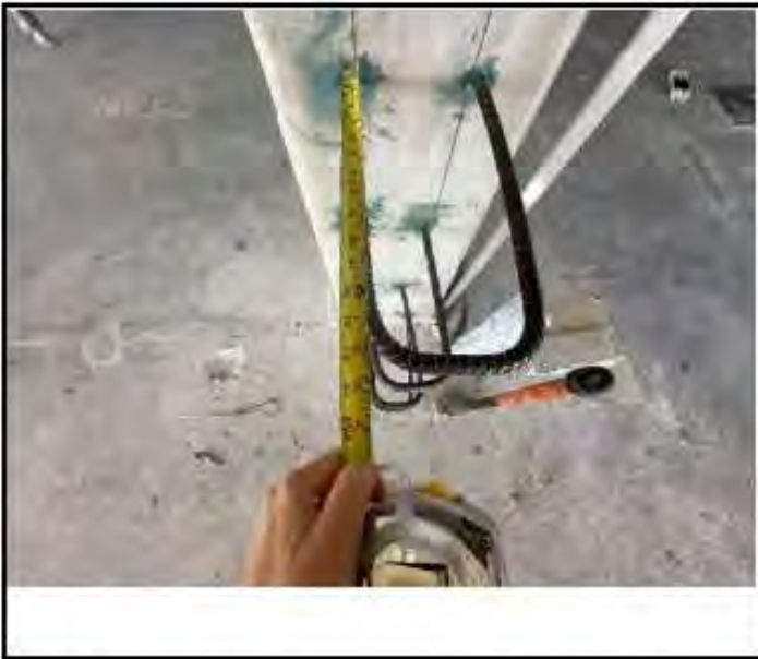
Figure 38. Photograph from Threshold Inspection Report No. 138 showing installed dowels on the north side of column J-2 part of the rectification of the column and roof structure.
