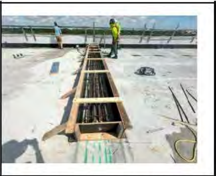
Figure 58. Photograph from Threshold Inspection Report No. 207 showing completed installation of reinforcement in in upturned beam.
