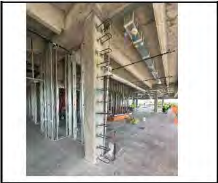
Figure 36. Photograph from Threshold Inspection Report No. 138 showing installed dowels on the north side of column I-2 part of the rectification of the column and roof structure.
