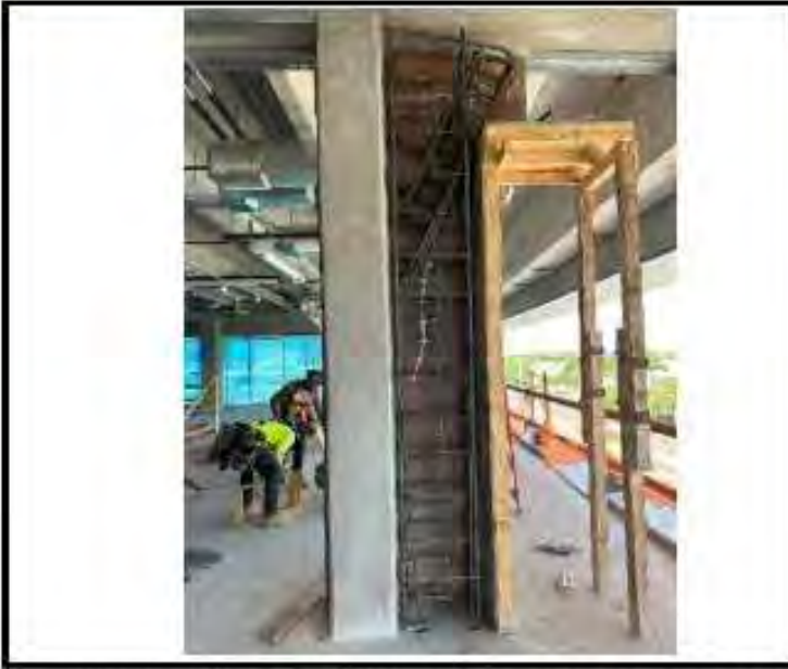
Figure 41. Photograph from Threshold Inspection Report No. 140 showing completed reinforcement installation at third story column enlargement.
