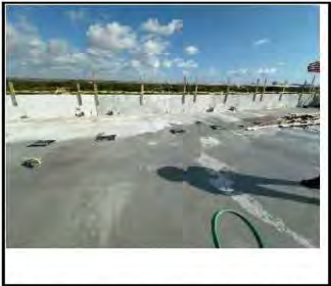
Figure 30. Photograph from Threshold Inspection Report No. 127 showing water which was sprayed onto the top of the roof slab at the north end of building.
