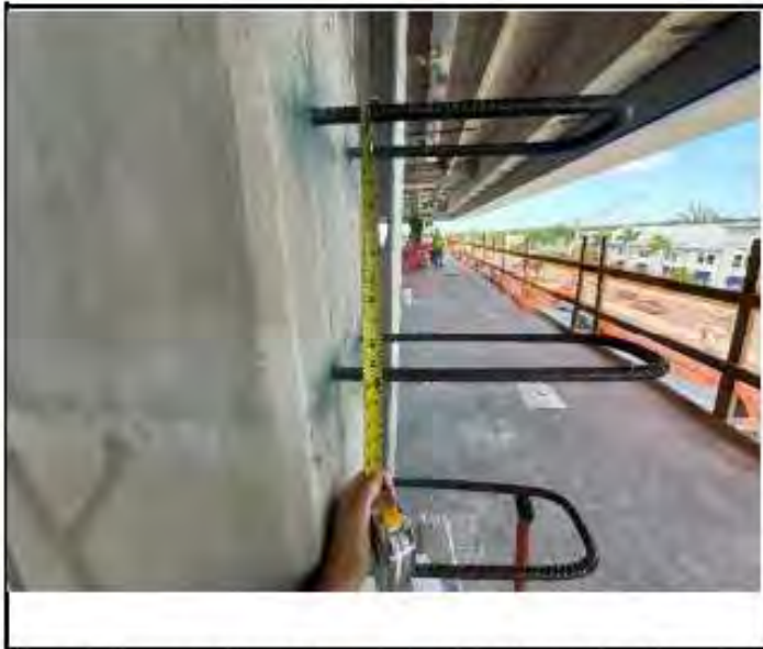
Figure 37. Photograph from Threshold Inspection Report No. 138 showing installed dowels on the north side of column J-2 part of the rectification of the column and roof structure.
