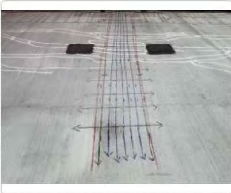
Figure 61. Photograph from ScanTek GPR report at Spot 3 (beams RSB-75 and RSB-76).
