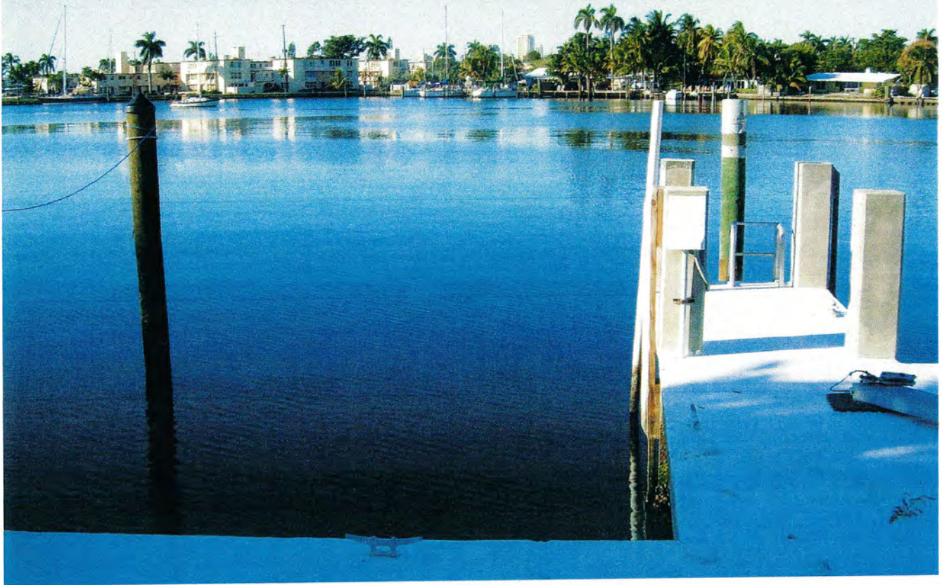
South end behind southern finger pier looking West over water
