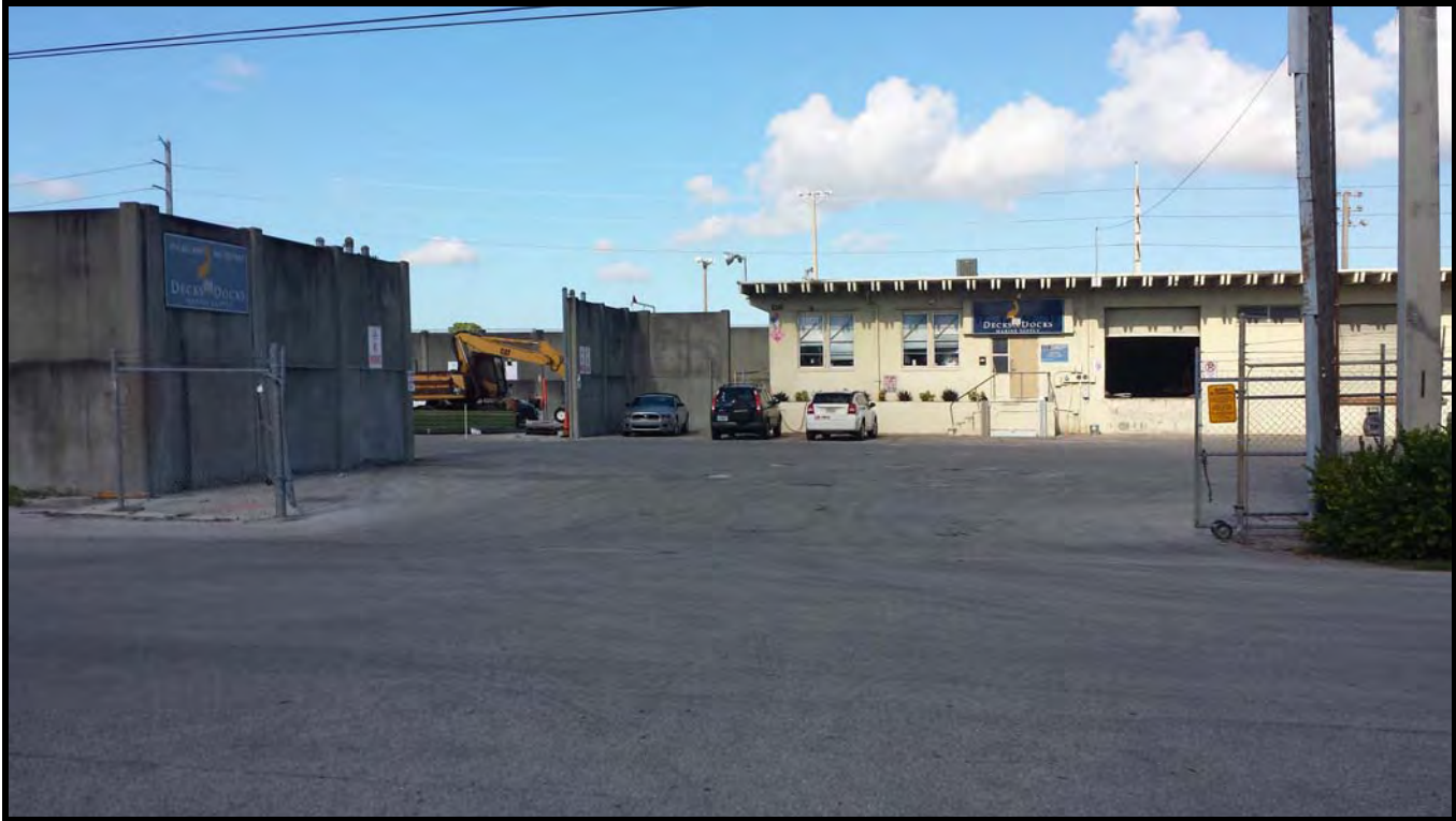
View of the northern most access point of the subject property along the west side of SW 1 st Avenue looking southwest.
