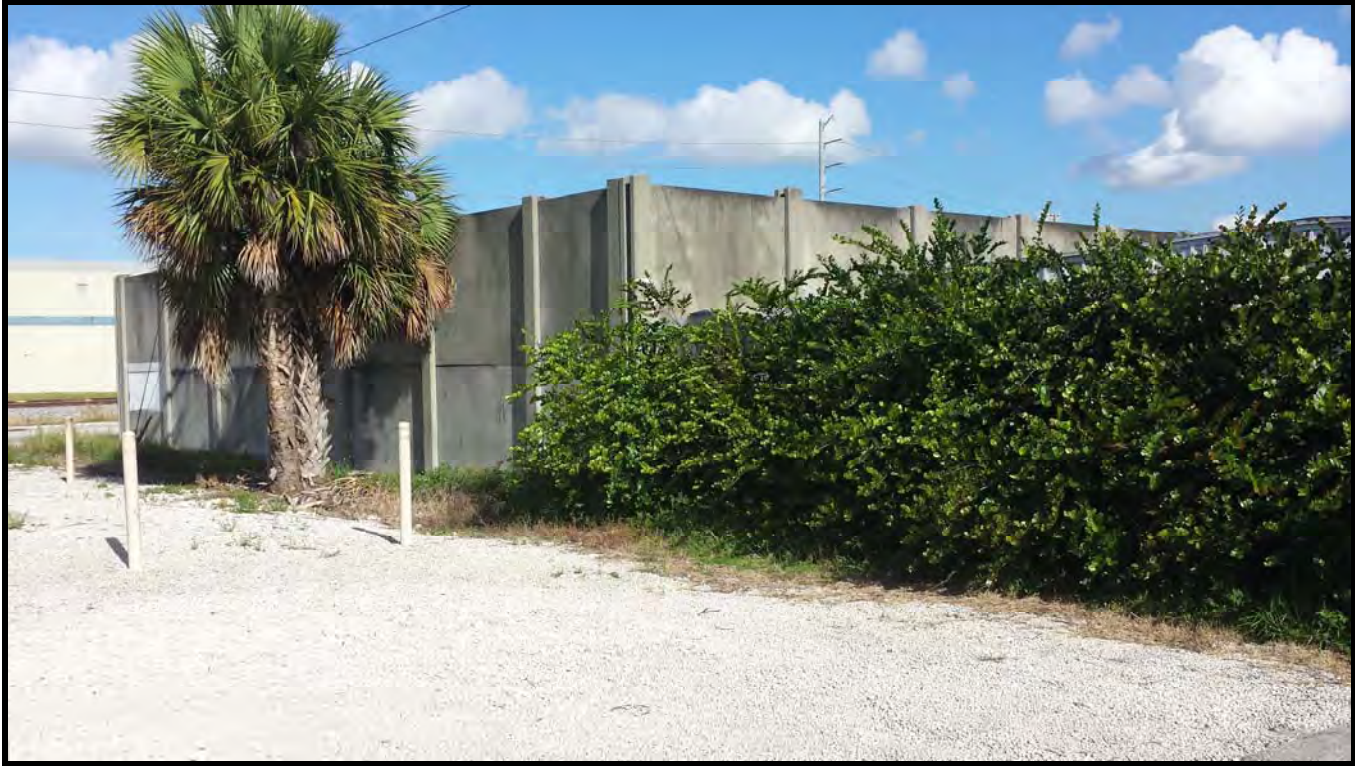
View of the southeast corner of the subject property looking northwest.
