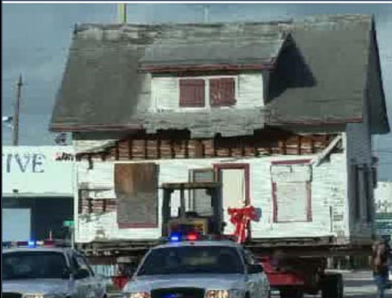
Crews move the historic Shippey House to its new location in Himmarshee Village. (Source: CBS4)
