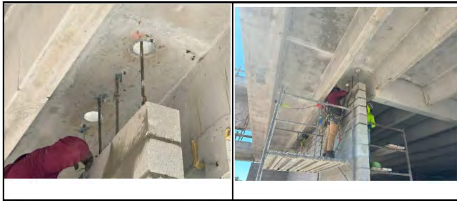
Figure 20. Photographs from Threshold Inspection Report No. 099 showing issue noted by inspector at top of "HQ Level 3 South CMU wall". Note PTA anchors and connection of vertical masonry bars to above slab in left image. Note that the bars are generally spliced to anchors attached to the slab with screws
