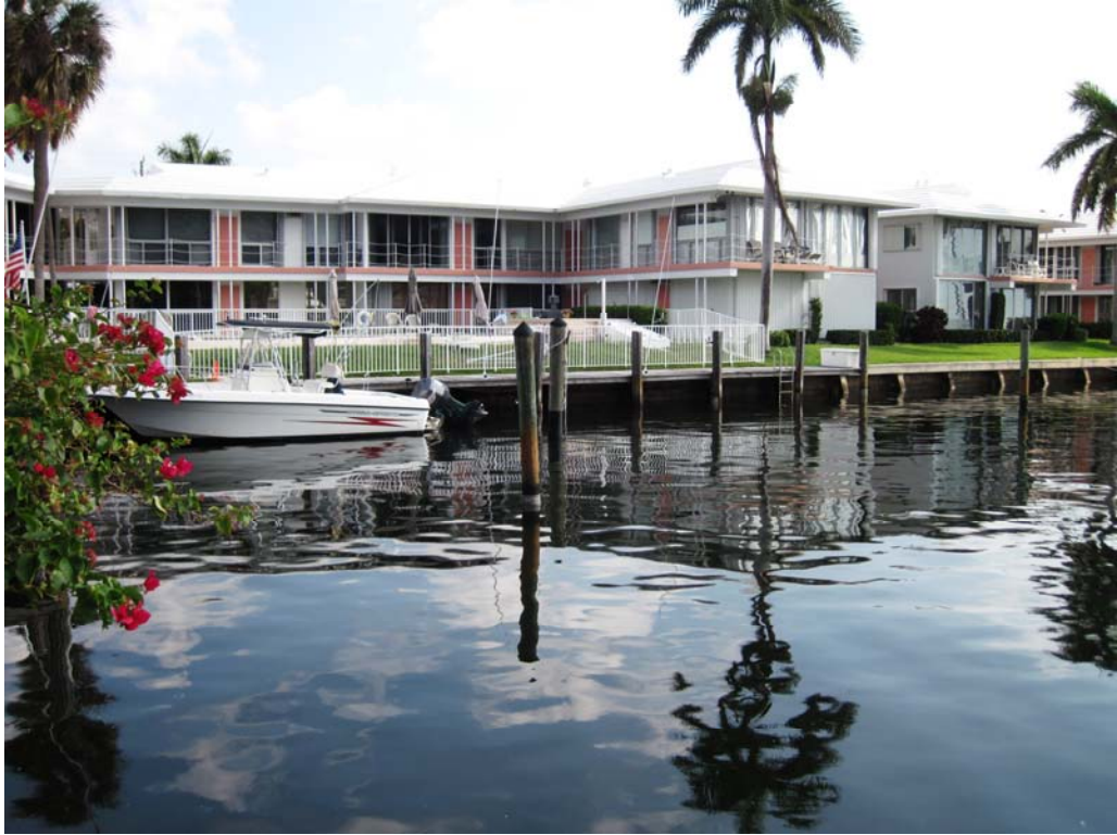
5. Northern property boundary, facing north.
