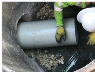
SSMH #5 - Short Module PP Pipe Insertion Through Manhole
