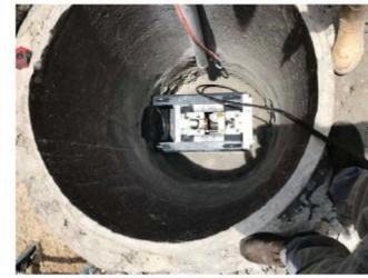
SSMH #55 - Static Pipe Bursting Rig Inside Manhole
