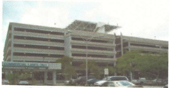
Ft. Lauderdale, City parking Garage
