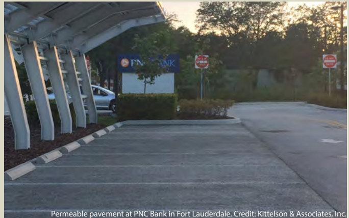
Permeable pavement at PNC Bank in Fort Lauderdale. Credit: Kittelson & Associates, Inc.
