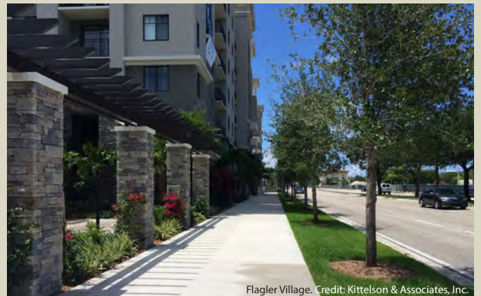
Flagler Village. Credit: Kittelson & Associates, Inc.
