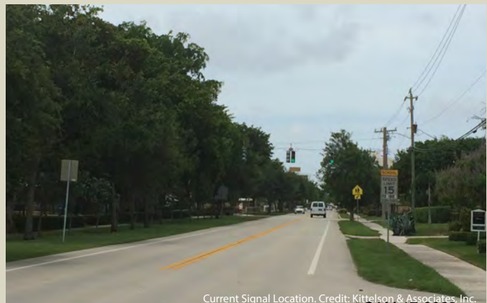
Current Signal Location. Credit: Kittelson & Associates, Inc.
