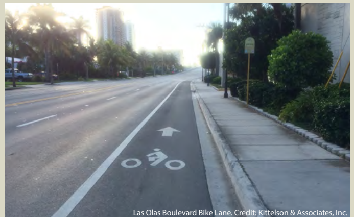
Las Olas Boulevard Bike Lane. Credit: Kittelson & Associates, Inc.
