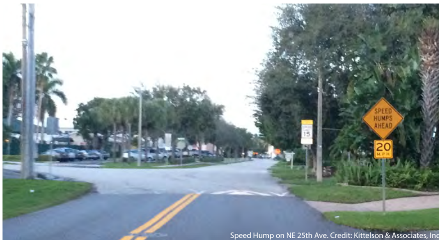
Speed Hump on NE 25th Ave. Credit: Kittelson & Associates, Inc.
