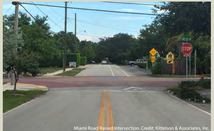
Miami Road Raised Intersection. Credit: Kittelson & Associates, Inc.
