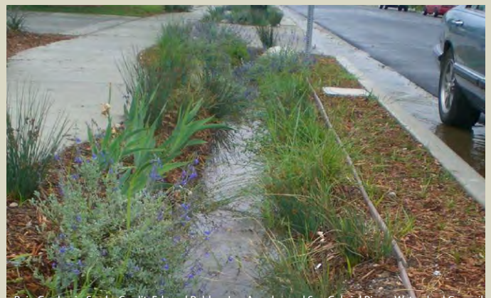
Rain Garden in Swale. Credit: Edward Belden, Los Angeles and San Gabriel Rivers Watershed Council
