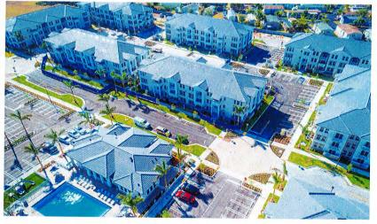
Alcazar Phase I Apartments, is the new construction of 9 buildings each 3 Stories in height. These buildings consist of 216 Walk Up Units. In addition to the 9 buildings, we are building a clubhouse and swimming pool, which will be reinforced with masonry and flat plate construction.
