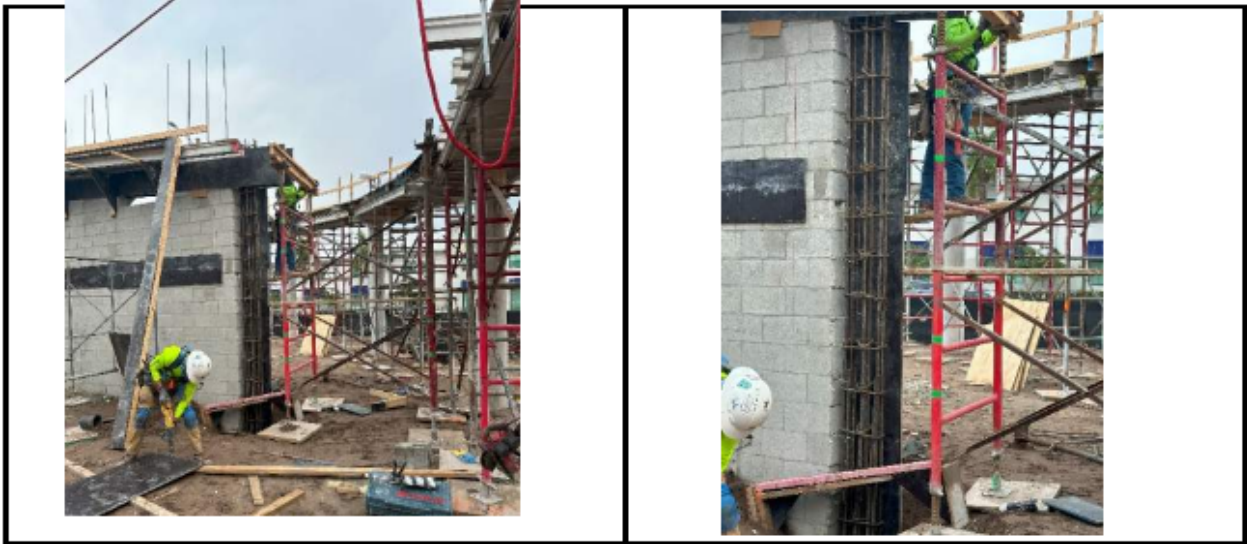
Figure 23. Photographs from Threshold Inspection Report No. 105 showing CMU wall in Area E under construction. Since the wall is being constructed prior to the roof structure, this CMU wall will take load from the roof structure as a bearing wall
