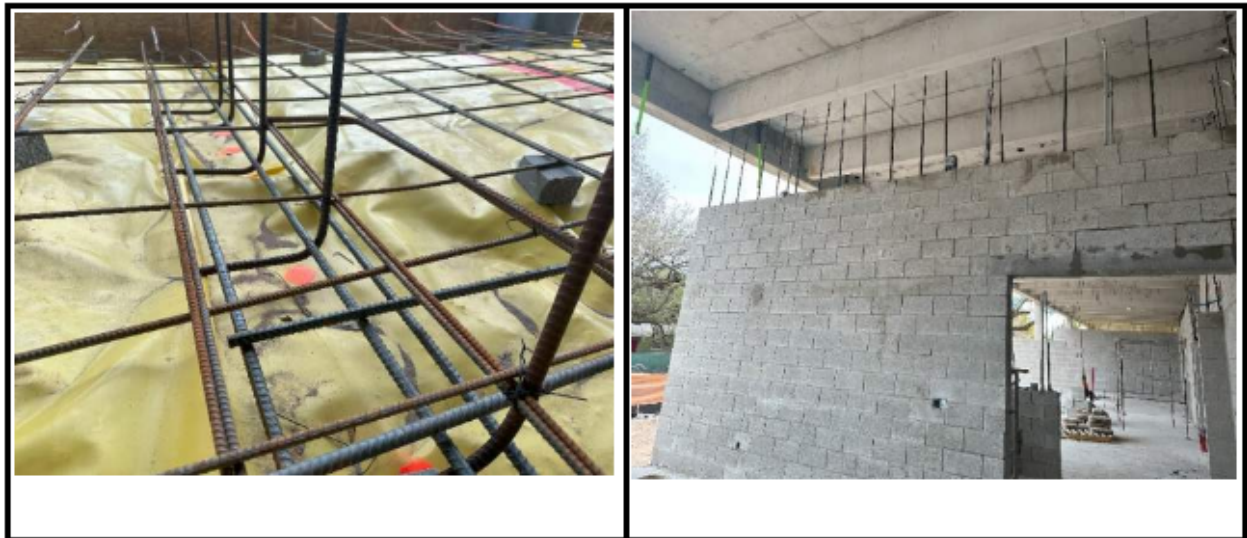
Figure 24. Photographs from Threshold Inspection Report No. 107. The photograph on the left shows hooked dowels at a thickened slab location under a wall. The inspector noted that the dowels needed to be shifted downwards. The photograph on the right shows a CMU wall in the first story under construction. Note that no shoring of the structure above is present, indicating that the CMU wall was not constructed as a bearing wall
