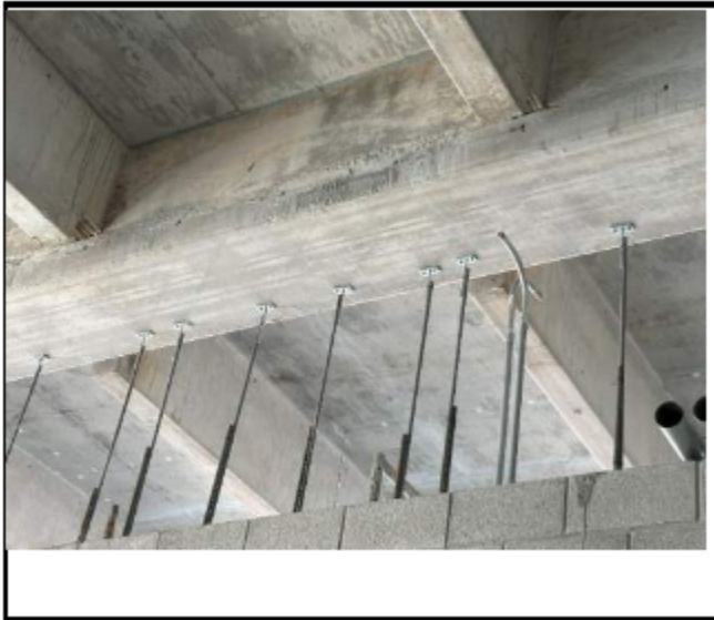
Figure 27. Photograph from Threshold Inspection Report No. 125 showing PTA connectors at bottom of soffit beam with the two screws attaching the plate of the anchor to the soffit beam
