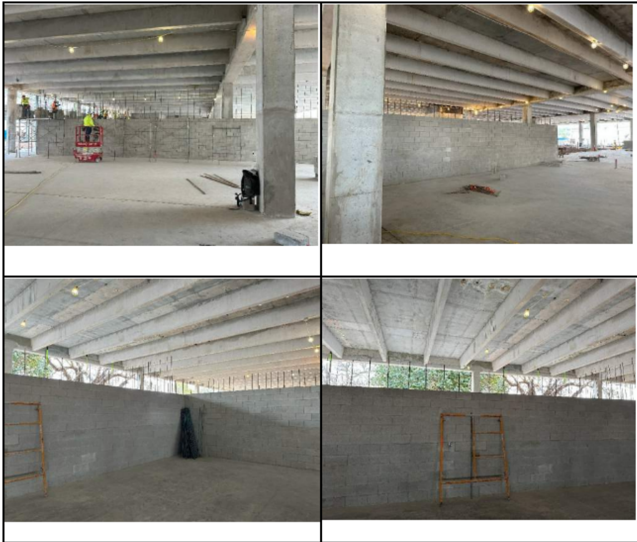
Figure 22. Photographs from Threshold Inspection Report No. 103 showing first story CMU walls under construction. Note the lack of shoring indicating that the CMU walls were not constructed as bearing walls
