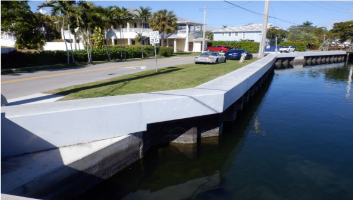
3. Central portion of the subject site, facing northwest.
