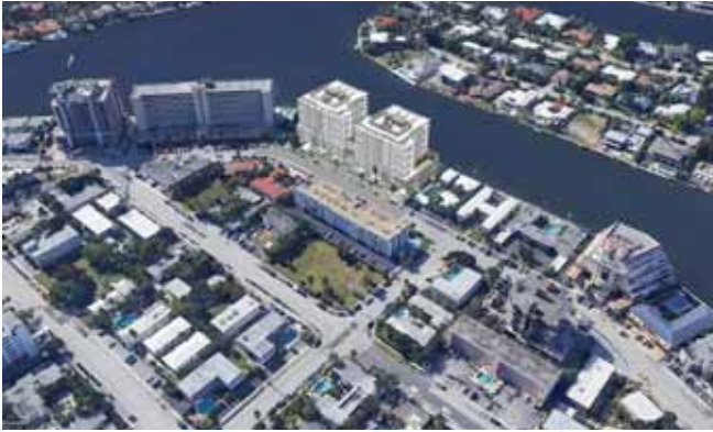
OBLIQUE VIEW - FROM THE NE
