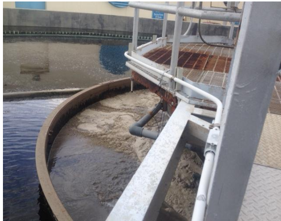
Existing walkway and platform
