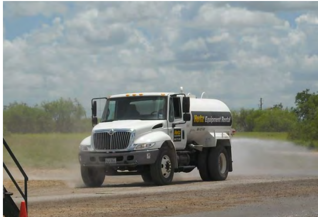
A water truck sprinkling to control dust on an access road.
