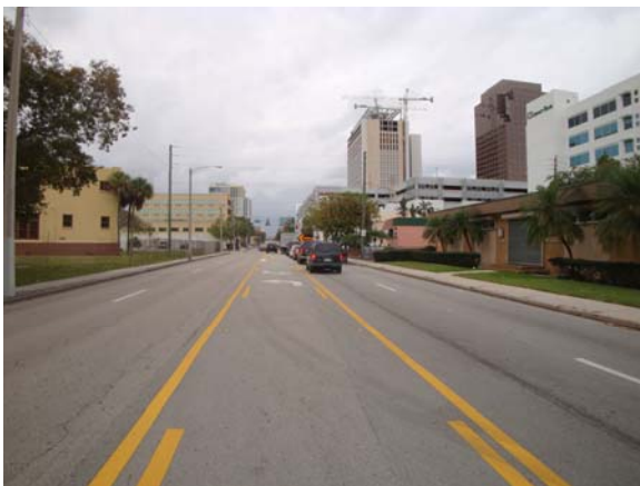
Subject Street Looking North
