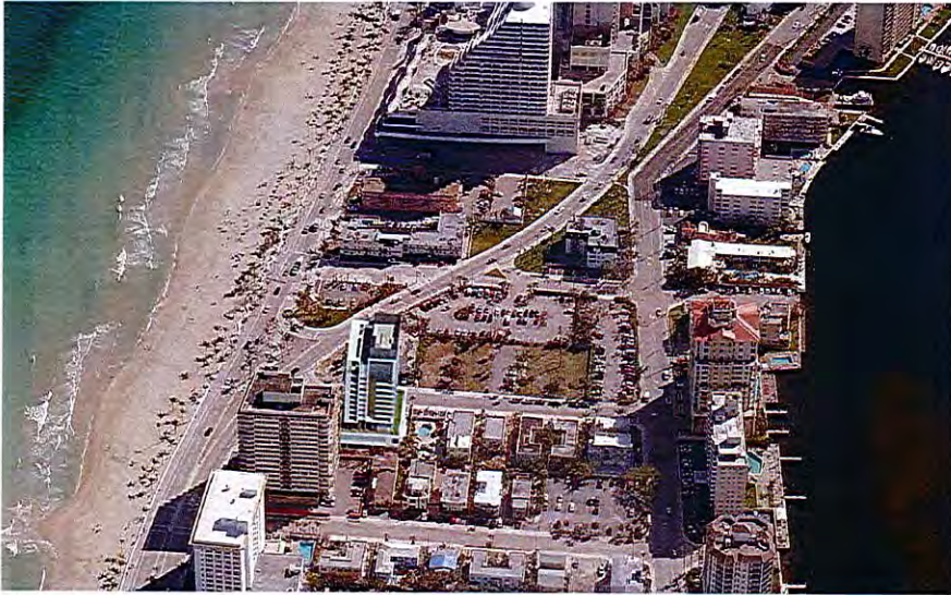
A1 AERIAL VIEW LOOKING SOUTH
