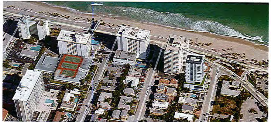
A4 AERIAL VIEW LOOKING EAST
