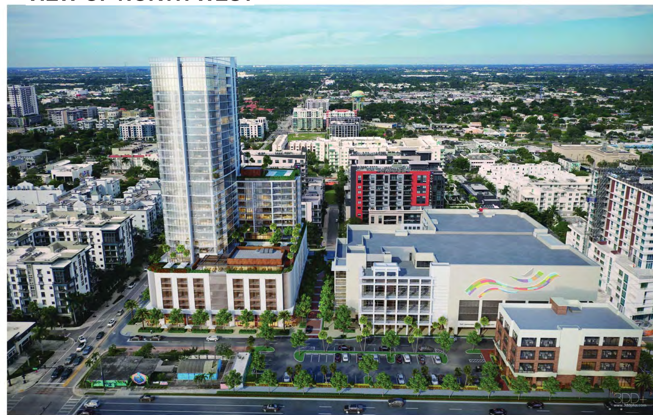
VIEW FROM EAST ABOVE FEDERAL HWY
