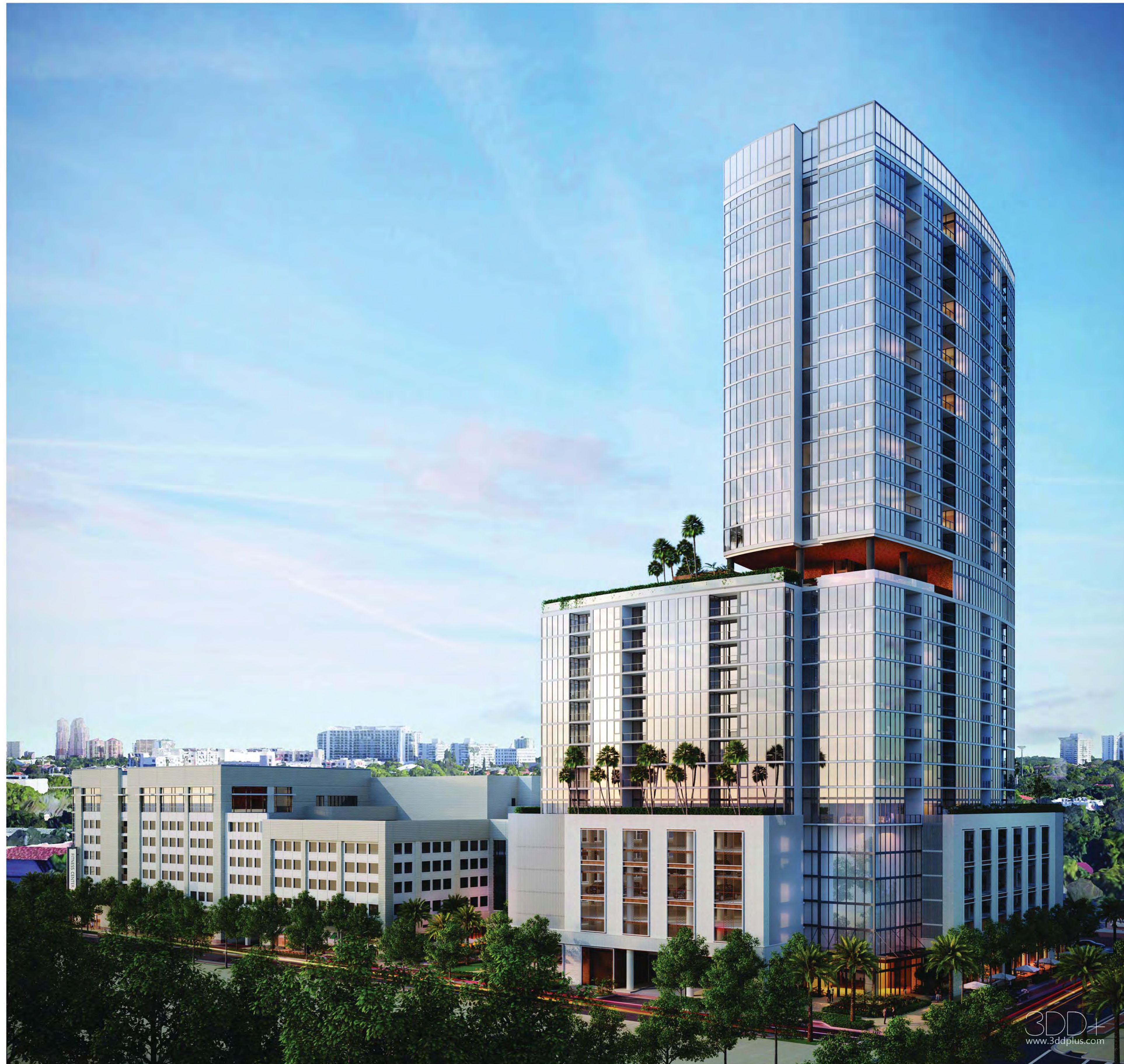
VIEW OF SOUTH WEST
