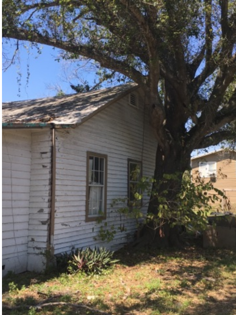
Side (East) Elevation of Existing House
