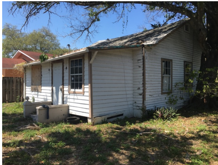
Front Elevation of Existing House, Facing South
