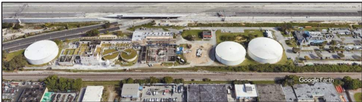
Figure #1: Fiveash Water Treatment Plant
