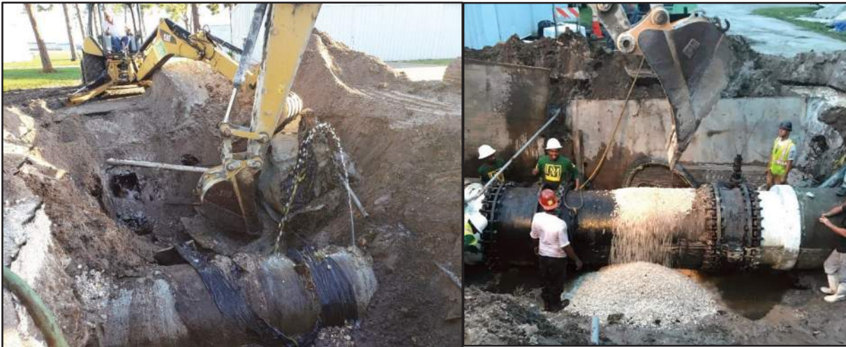
Figure #2: DMSI mobilized and completed repair of 42-inch raw Water main break in day one (Prospect Wellfield)
