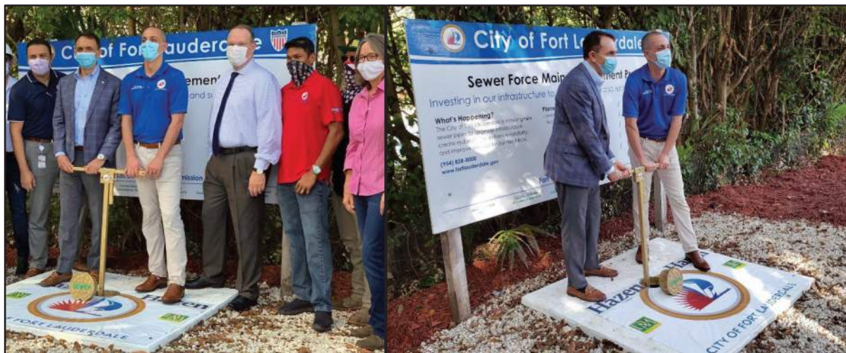
Figure #3: City Commission Activating the 54-inch Emergency Redundant Sewer Line installed by DMSI
