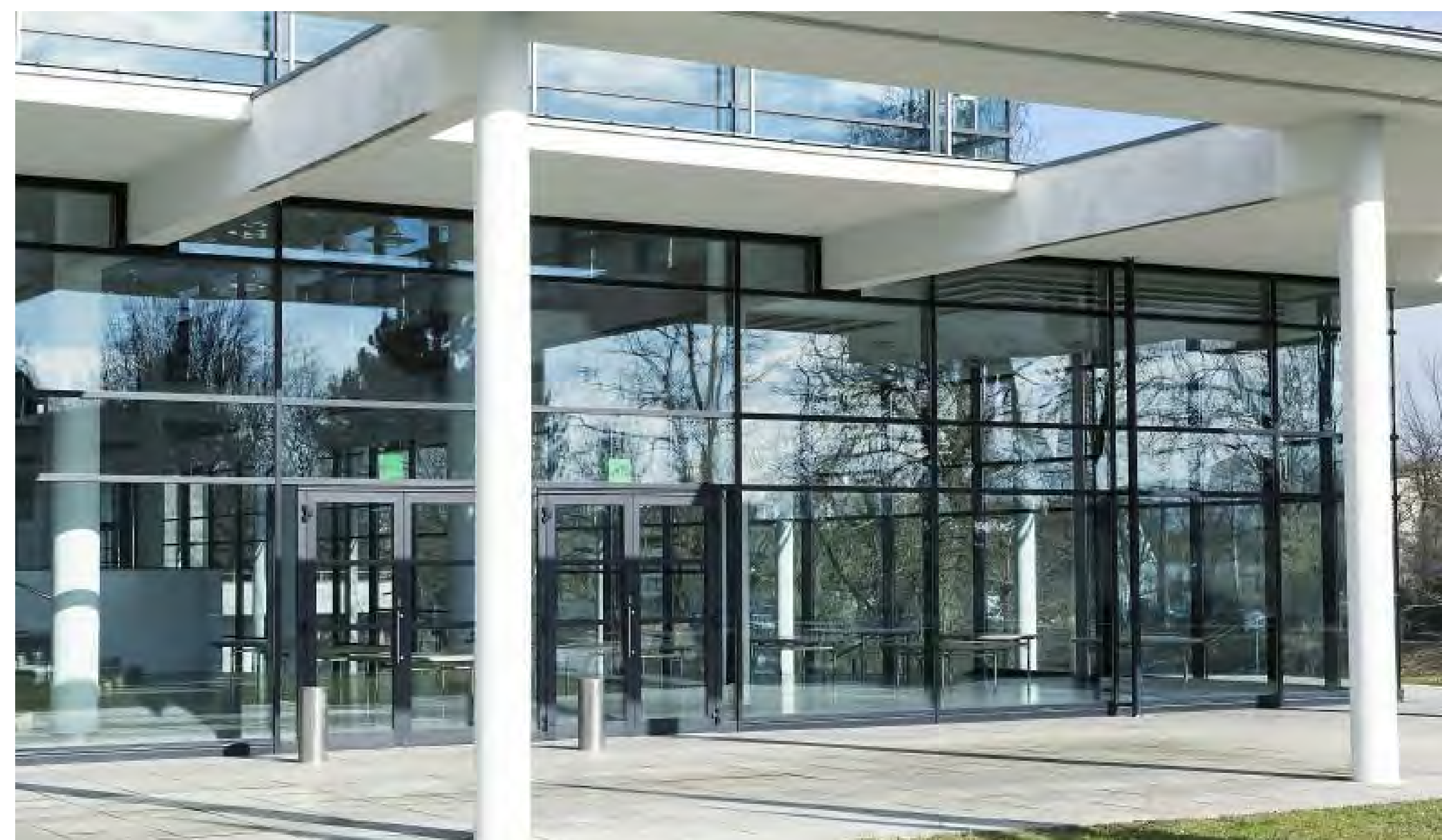
A. GLASS STOREFRONT NOTE: GROUND FLOOR GLASS TO BE THE CLEAREST POSSIBLE PERMITTED BY THE FBC.
