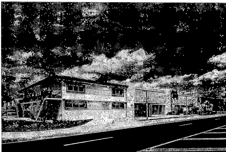
In 2016, Gurrimate completed the restoration and adaptive reuse of the Historic Hampton House with O'Donnell & Naccarato (formerly Douglas Wood & Associates) and Laura Llerena & Associates. This historic preservation project received numerous awards including from AIA Miami, AIA Florida, and Dade Heritage Trust.
