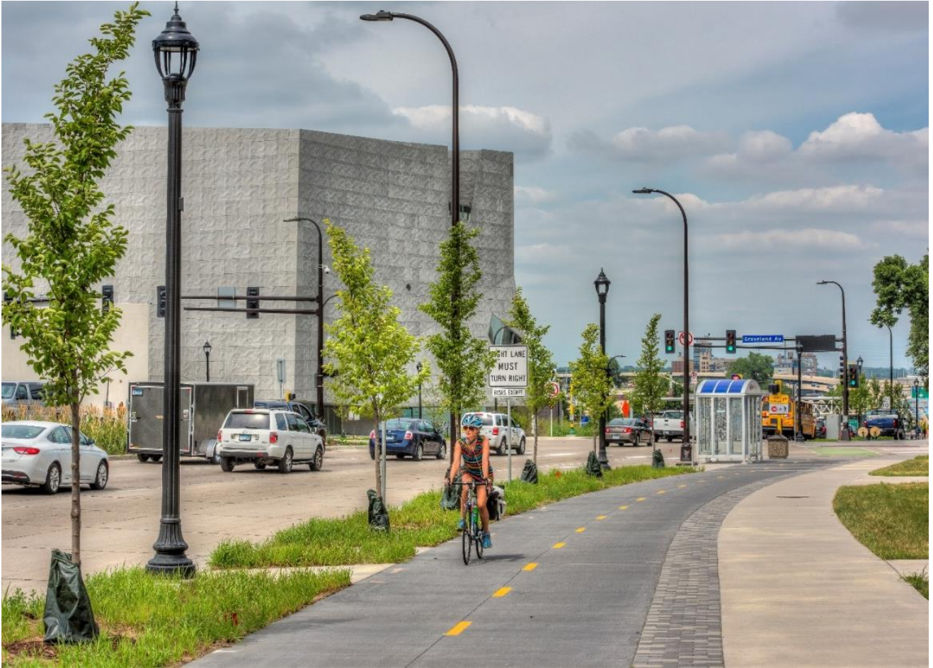
Photo Credit: Kimley-Horn, Minneapolis (Two-Way Raised Separated Bicycle Lanes)
