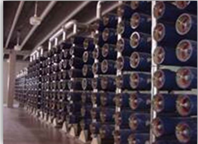
Sawgrass Nano Filtration WTP, City of Sunrise – MWH designed the system and vessels such that the low pressure nanofiltration process could be upgraded to a high pressure Reverse Osmosis and vice versa with minimum process changes.
