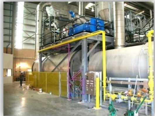
The MWH project team designed a new centrifuge dewatering and thermal drying facility for Hillsborough County, which now allows the County to sell its pelletized biosolids product to regional growers as a fertilizer.
