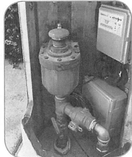
EchoShore-TX node integrated into an above ground chamber in Las Vegas
