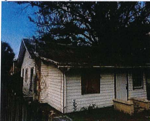
Figure 3 Left Side View of Existing House to be Demolished
