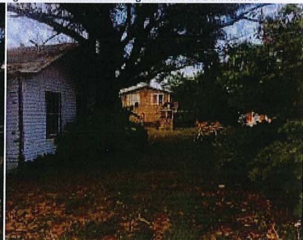
Figure 4 Right Side View of Existing House to be Demolished
