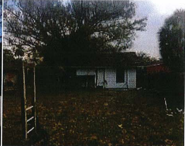
Figure 2 Back View of Existing House to be Demolished
