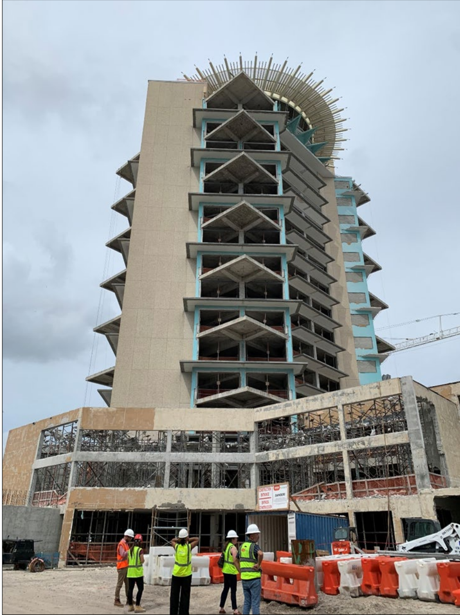
Figure 9. Pier 66 Hotel Tower. Southeast building perspective, camera facing northwest. Photograph taken October 18, 2022.
