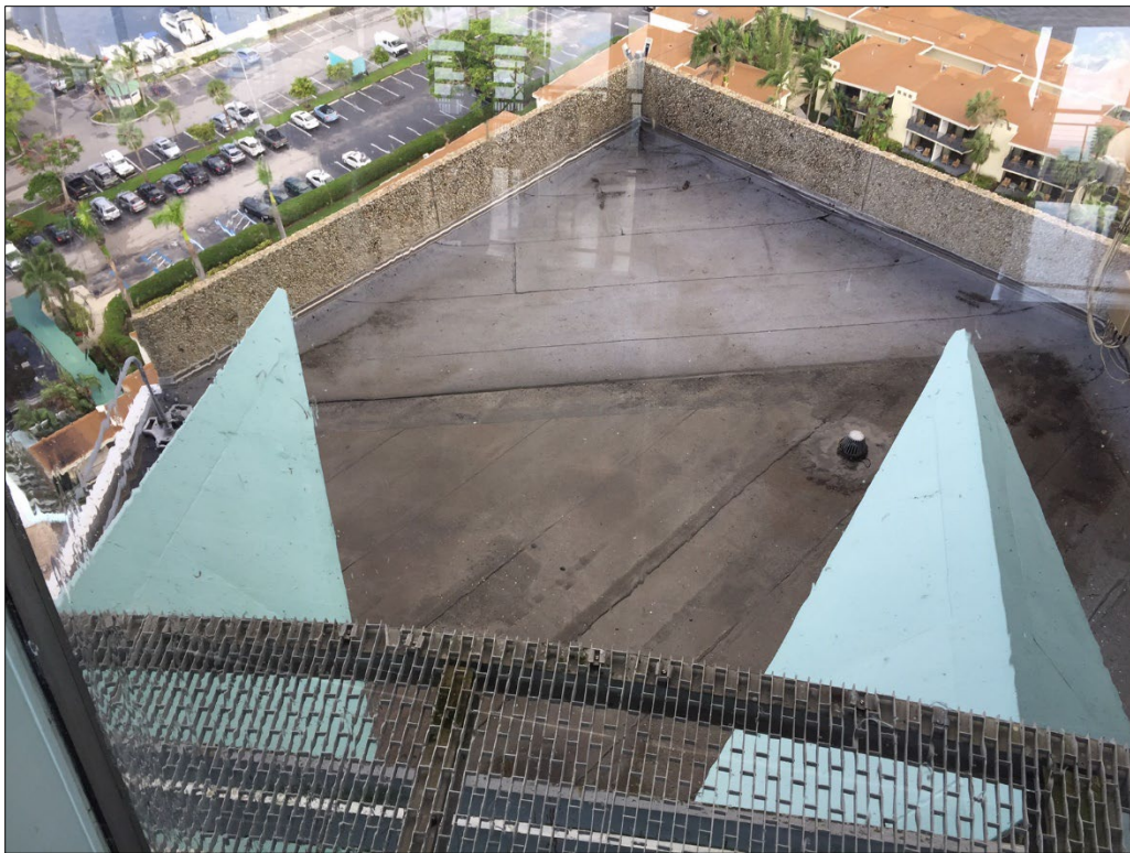
Figure 7. Pier 66 Hotel Tower. Trihedrons. Camera facing down and northwest. Photograph taken October, 2017.
