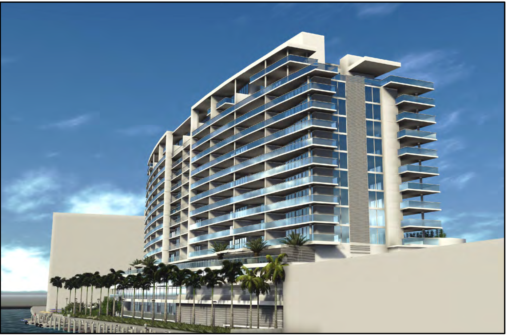
WATERWAY - OVERALL VIEW LOOKING SOUTH
