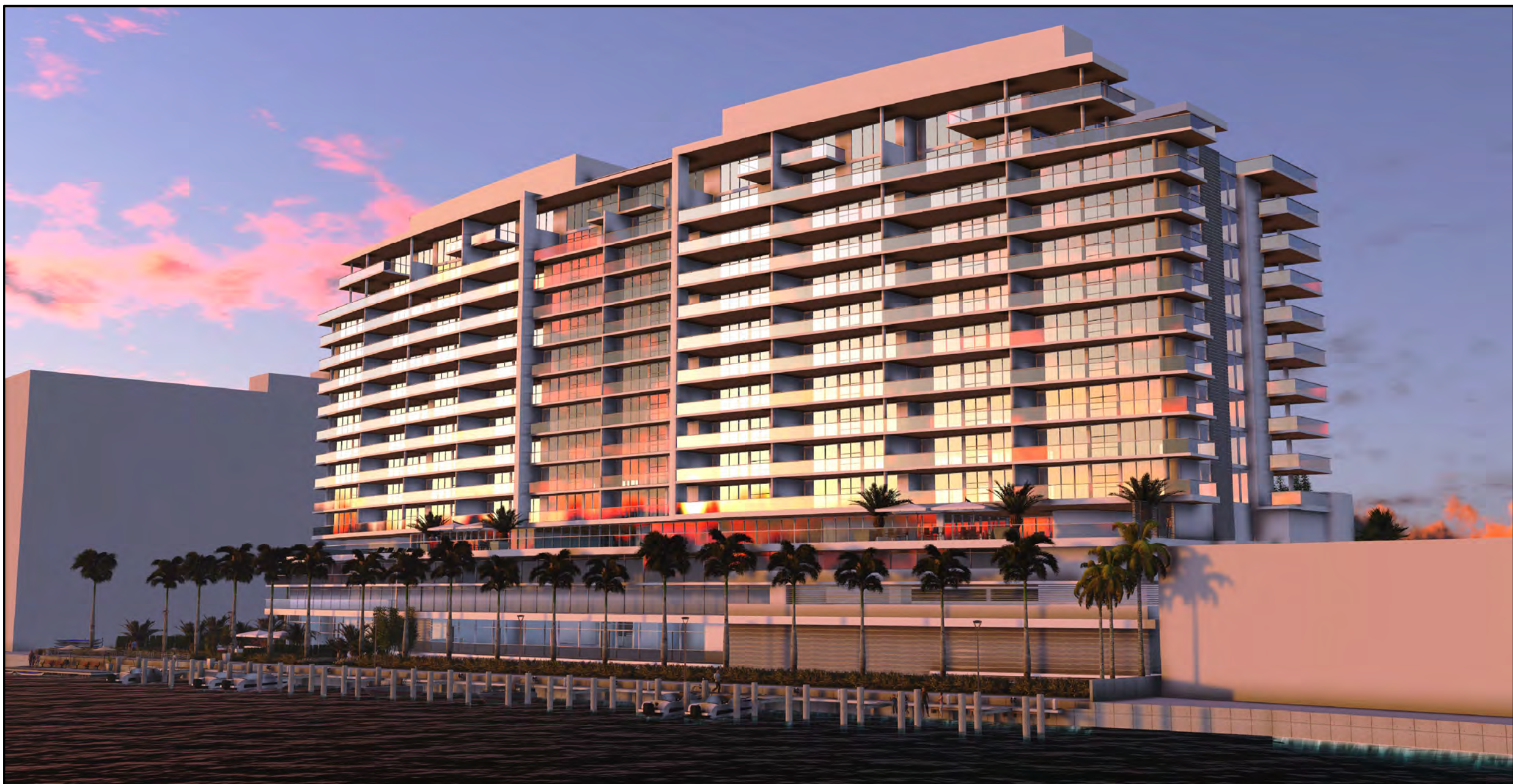
VIEW LOOKING SOUTH WEST
