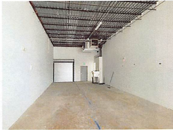
Typical Vacant Bay
