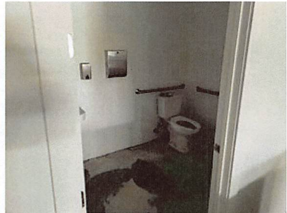
Vacant Bay Bathroom
