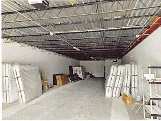
Typical Vacant Bay
