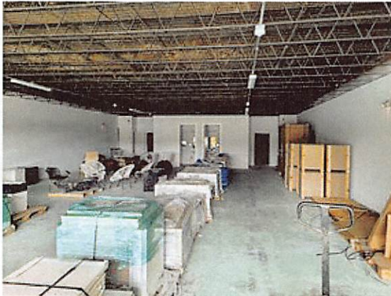
Typical Vacant Bay
