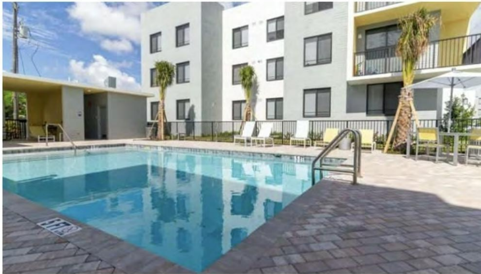
Palm Beach County Housing and Economic Development Department announced that Berkeley Landing Apartments marked a milestone with the grand opening of its new 112-unit multi-family residential community located at 3100 Broadway in Riviera Beach. (Palm Beach County Housing and Economic Development Department)
