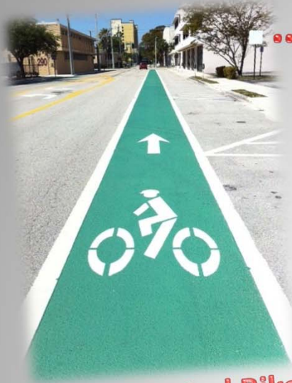
Painted Designated Bike Lane (NE 3rd Street)
