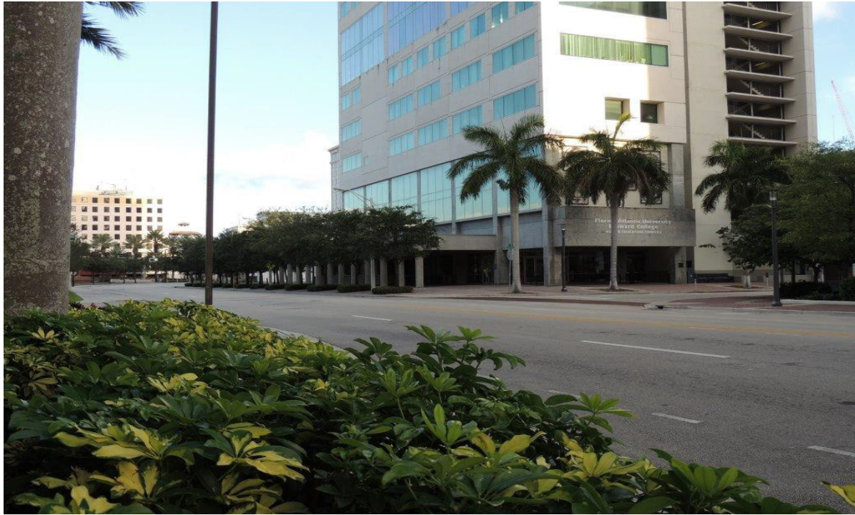
BCC/FAU Tower on Las Olas - 1995 blends Tree/Palm requirement but would not meet the 75% Increase in Shade Tree Percentages.
