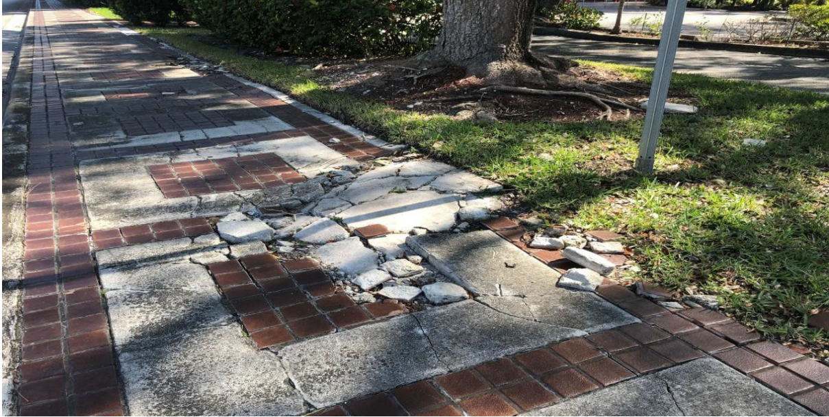
The location of the increase of Shade Trees in the requirements will jeopardize the sidewalks and adjacent infrastructure with or without the use of Structural Soil or root barriers.
