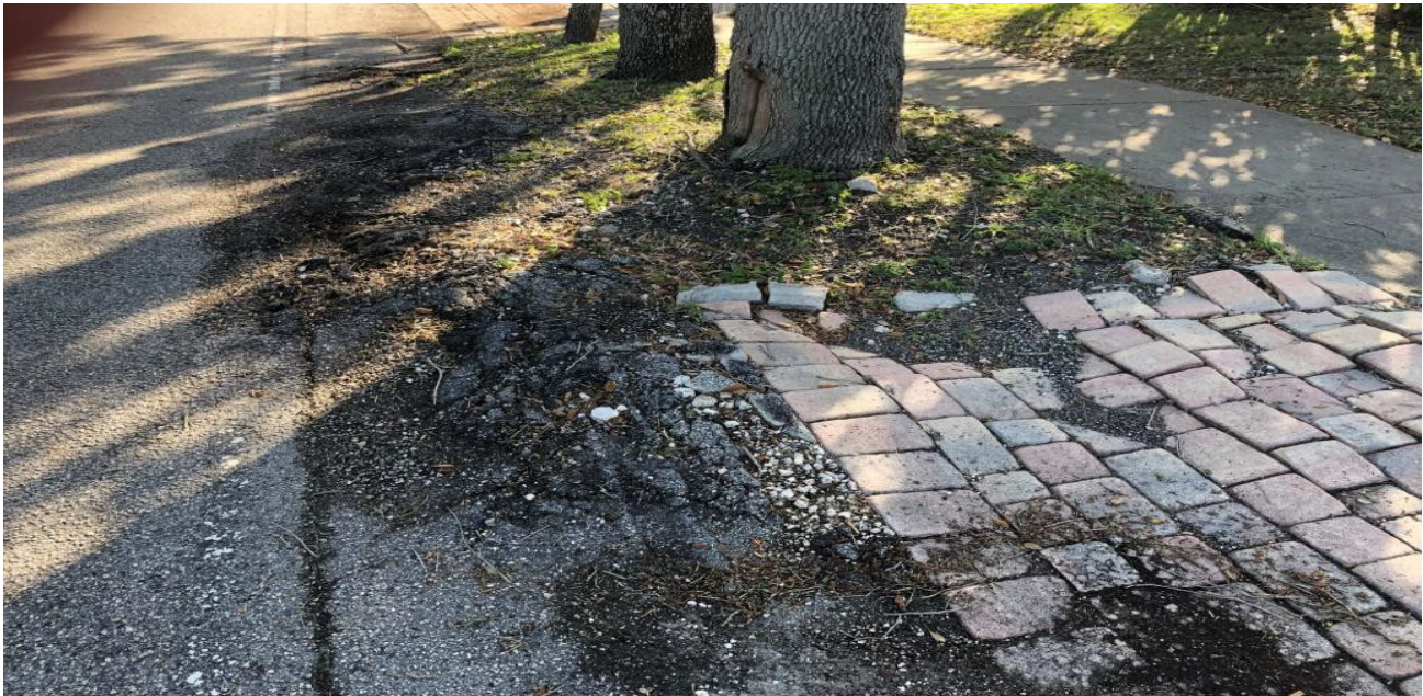
Many times, trees are planted in the wrong place or are the selection of an inappropriate species which leads to.....Costly Repairs.
