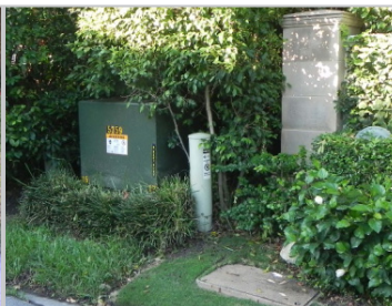
Single phase transformers and AT&T/Comcast service pedestals
