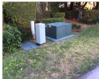
Single phase transformers and AT&T/Comcast service pedestals
