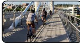
Bridge Multi-Use Paths
