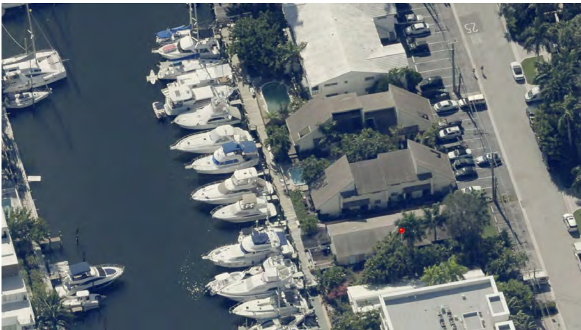
2. Northern portion of the subject site, facing south along the Rio Grande Waterway.
