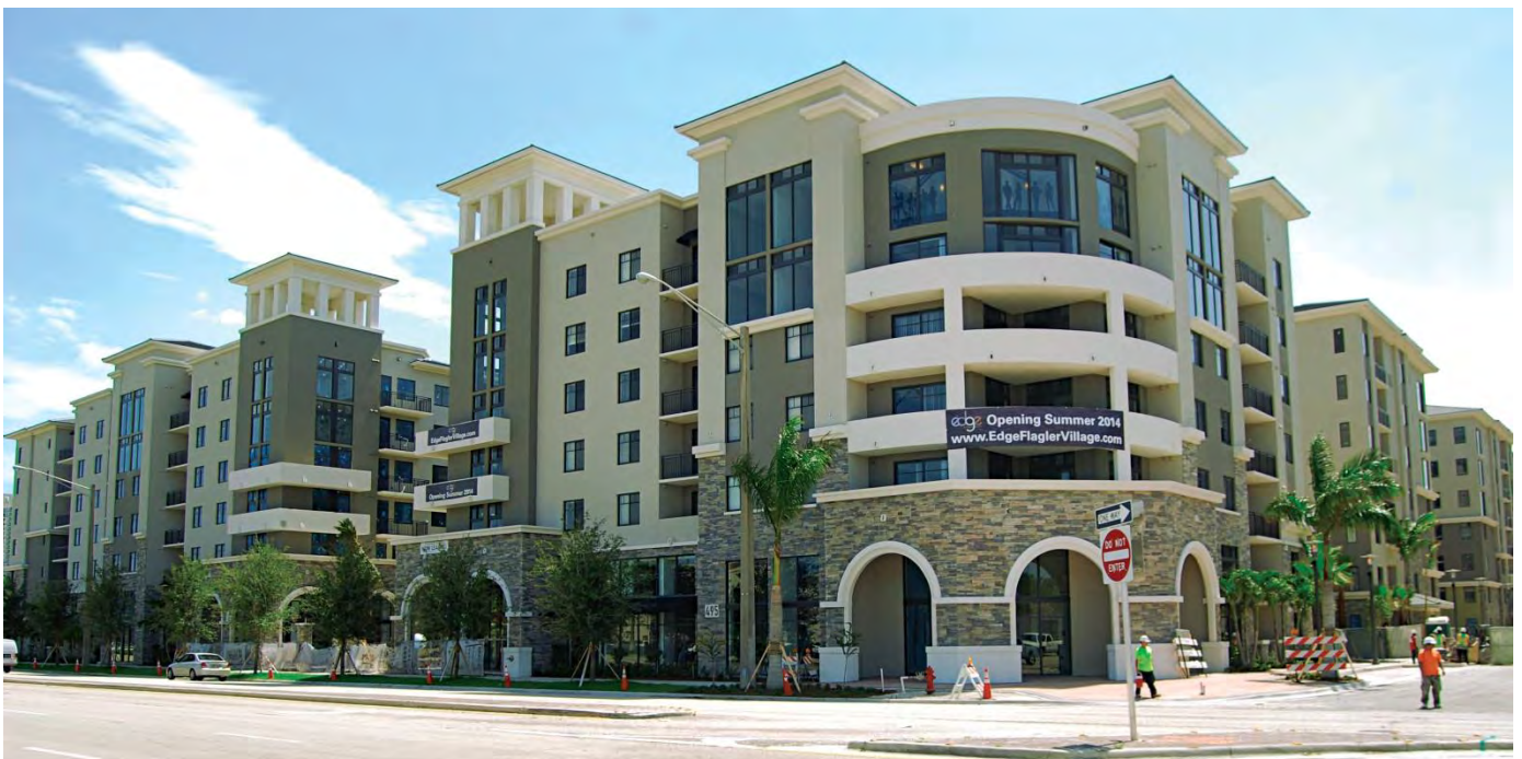
The Edge at Flagler Village, a new residential development in Downtown Fort Lauderdale
