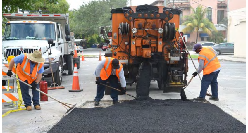
Public Works crew completing hot-in-place asphalt patching
