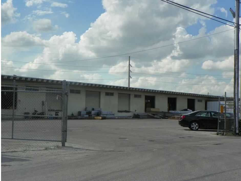
View of warehouse portion of the improvements at north end of site
