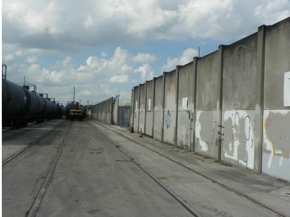
View of western boundary line along the FEC railroad right of way
