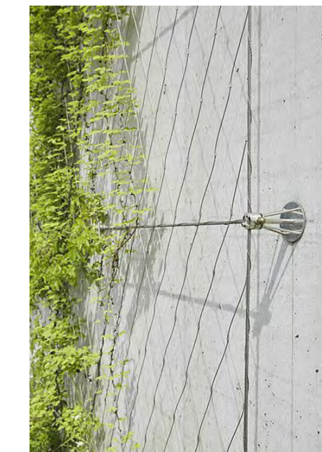
2 GREEN SCREENS HARDWARE Scale: NTS
