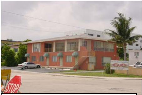
NW corner of Riomar Street and Birch Road 2-story residential
