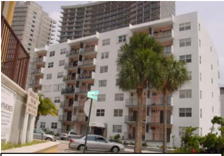
3000 Riomar Street 7-story condominium
