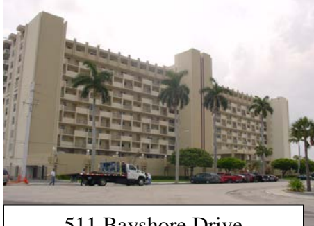
511 Bayshore Drive 11-story condominium
