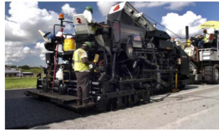
Figure 3 - Conventional Cold Mill & Overlay Construction
