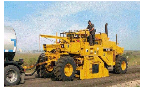
Figure 4 - Full Depth Reclamation (FDR) Base
