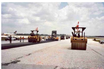
Figure 5 - Completed ARMI at Time of Test Section Construction
