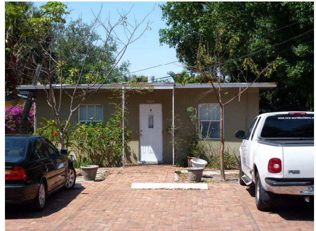
17 Adjacent Property to the east, North side of Coontie Court from Street Frontage (1225 Coontie Court)
