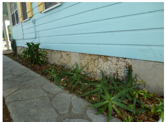
6 Residence 'A' - Coral Rock Filler in Foundation
