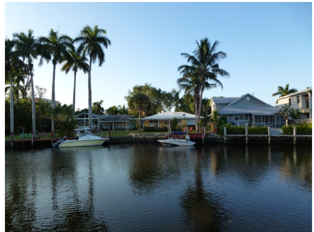
5 Residence 'A' – Right Side (South) Elevation – River Frontage
