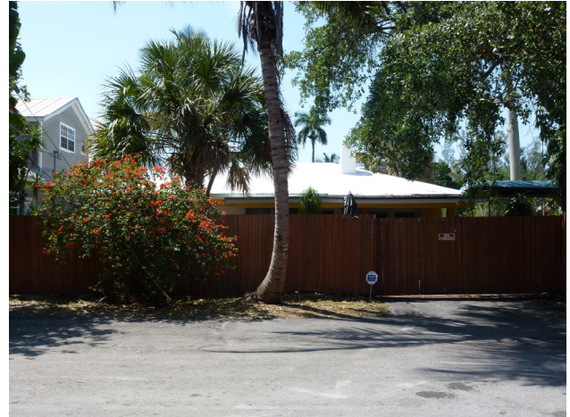
16 Adjacent Property to the East – South Side of Coontie Court from Street Frontage (1224 Coontie Court)
