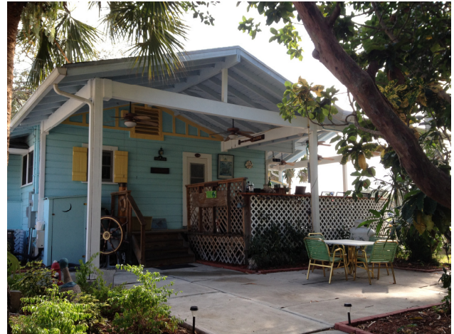
4 Residence 'A' – Rear (West) Elevation
