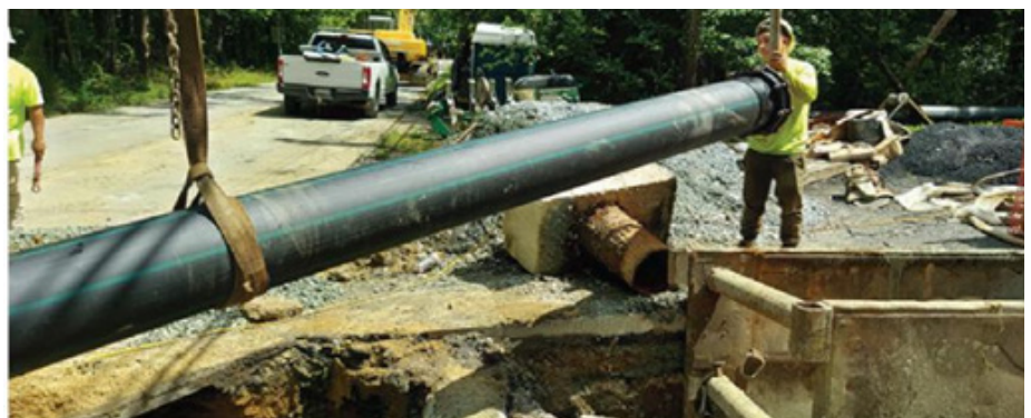
Rigging HDPE in place at pump station
