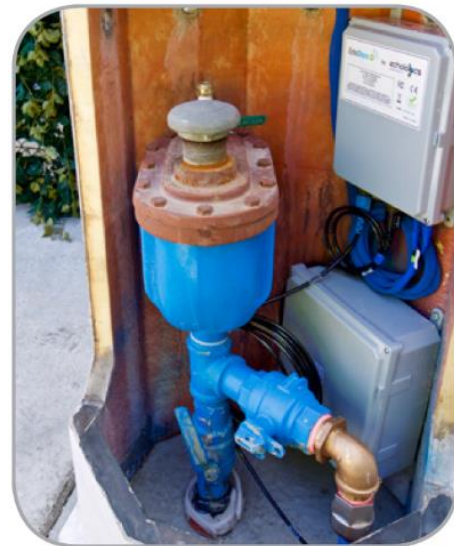
EchoShore-TX node integrated into an above ground chamber in Las Vegas
