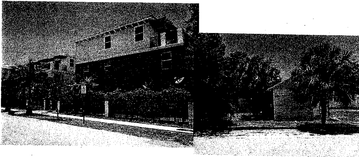
West of site along Arpeika Street
