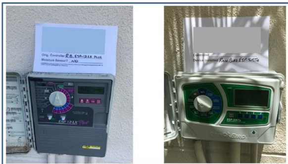
Figure 2a. A typical controller replacement under the NIS's 'Smart' Irrigation Technology Deployment Program. Antiquated clock timers (shown at left) are replaced with state-of-the-art digital controllers and on-site weather sensors (photo at right).
