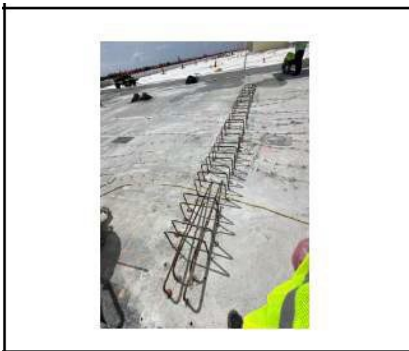
Figure 56. Photograph from Threshold Inspection Report No. 202 showing installed inverted "U" shaped stirrups and end "L" bars in upturned beams.
