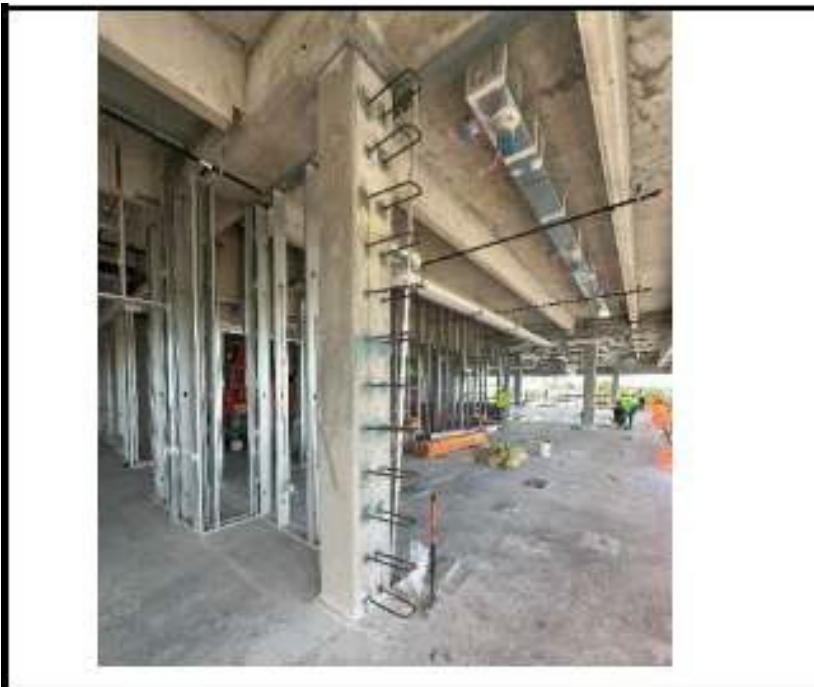
Figure 36. Photograph from Threshold Inspection Report No. 138 showing installed dowels on the north side of column J-2 part of the rectification of the column and roof structure.
