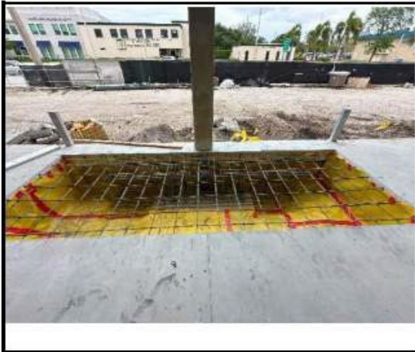
Figure 49. Photograph from Threshold Inspection Report No. 142 showing completed reinforcement placement at column footing enlargement.
