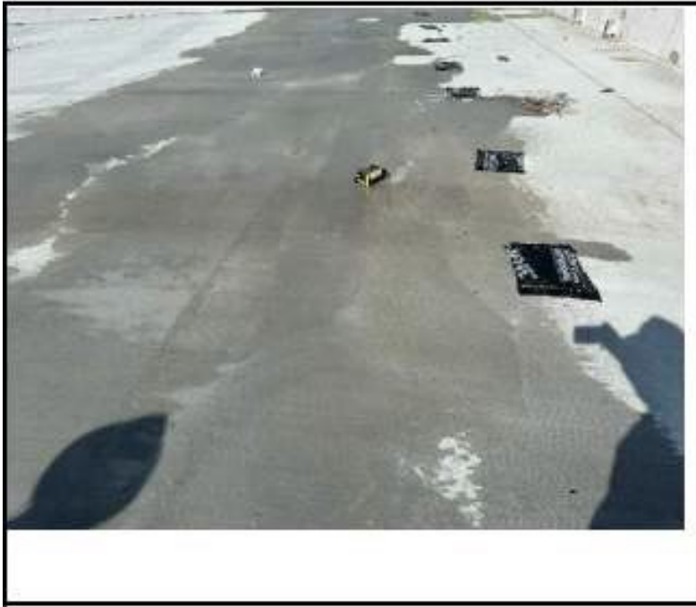
Figure 29. Photograph from Threshold Inspection Report No. 127 showing water which was sprayed onto the top of the roof slab at the north end of building.
