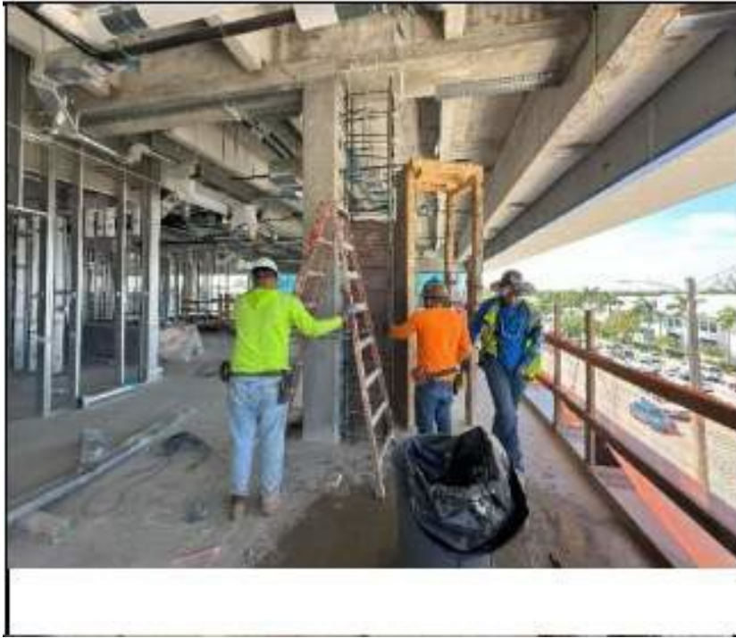
Figure 39. Photograph from Threshold Inspection Report No. 139 showing installed vertical reinforcement and horizontal ties at third story column enlargement.
