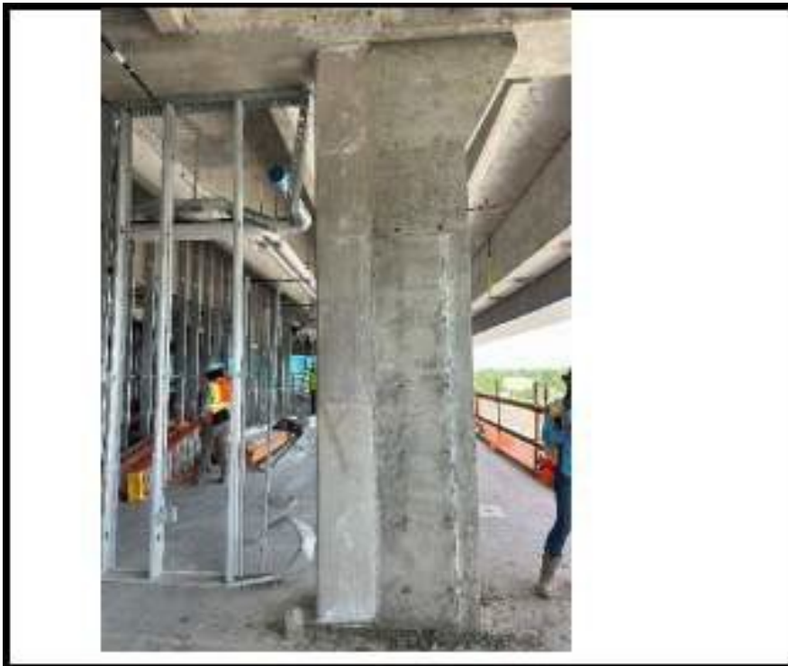
Figure 46. Photograph from Threshold Inspection Report No. 141 showing completed column enlargement.
