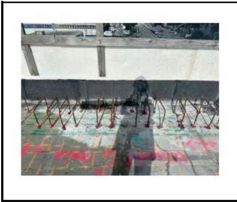
Figure 55. Photograph from Threshold Inspection Report No. 202 showing installed inverted "U" shaped stirrups in upturned beams.
