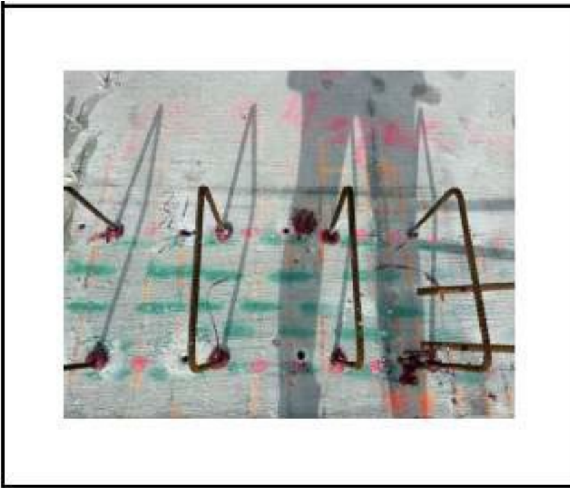
Figure 53. Photograph from Threshold Inspection Report No. 201 showing installed inverted "U" shaped stirrups in upturned beams.
