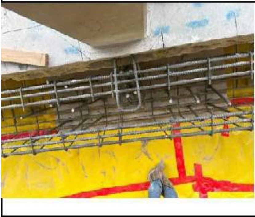
Figure 47. Photograph from Threshold Inspection Report No. 141 showing continuing work on column footing enlargement.
