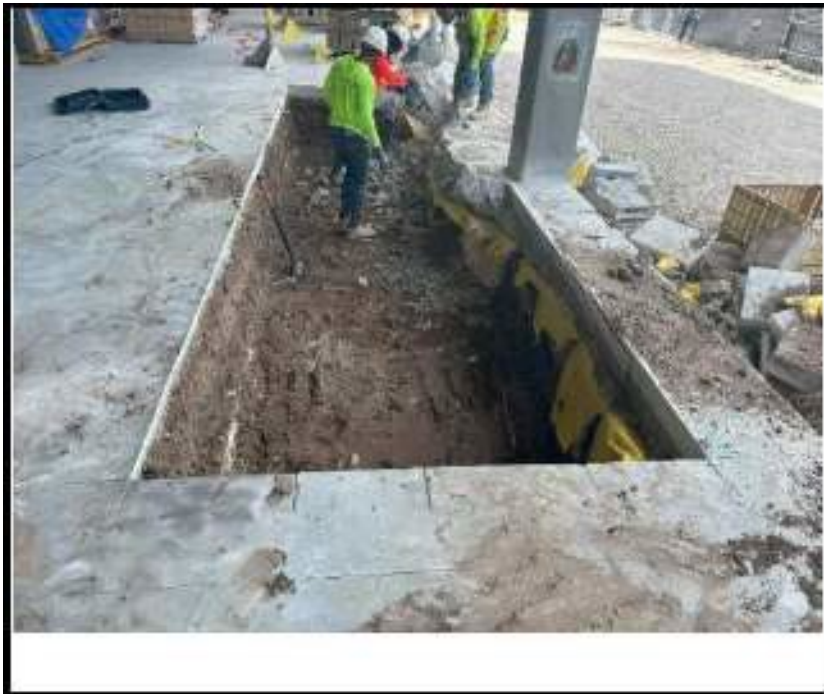
Figure 40. Photograph from Threshold Inspection Report No. 139 showing work to enlarge the footing at the base of either column H-2 or J-2.
