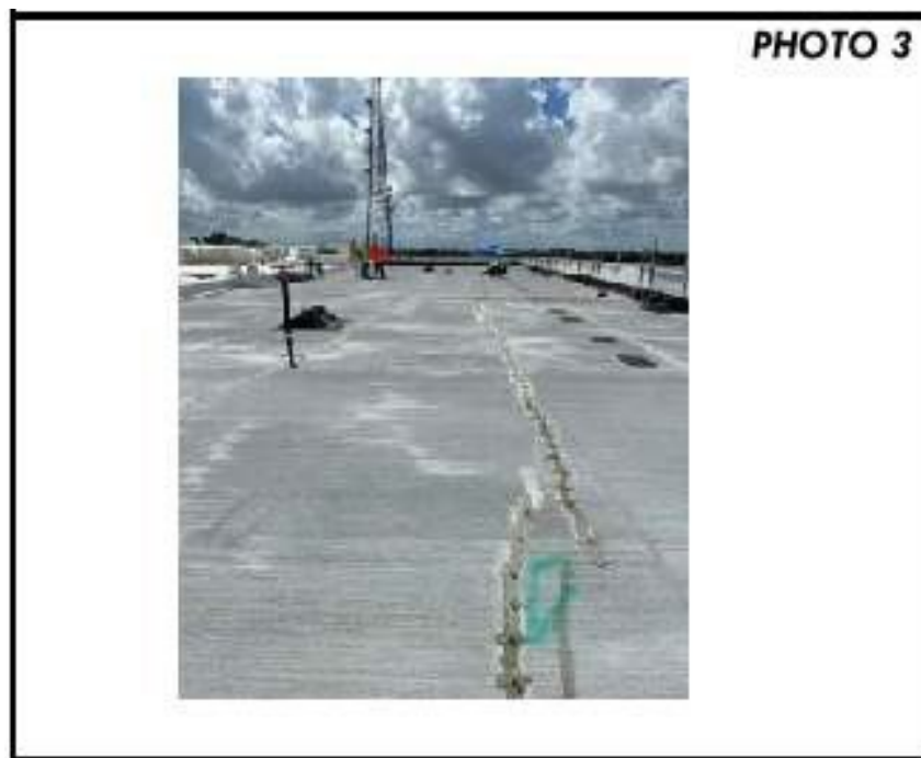
Figure 52. Photograph from Threshold Inspection Report No. 200 showing crack preparation and injection ports for epoxy injection of cracks in roof slab.
