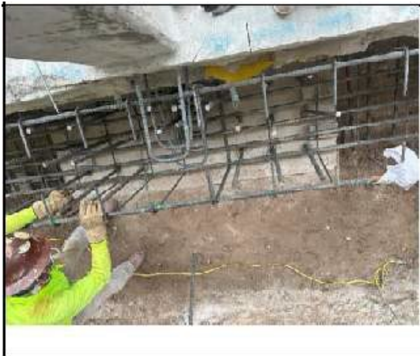
Figure 48. Photograph from Threshold Inspection Report No. 141 showing continuing work on column footing enlargement.
