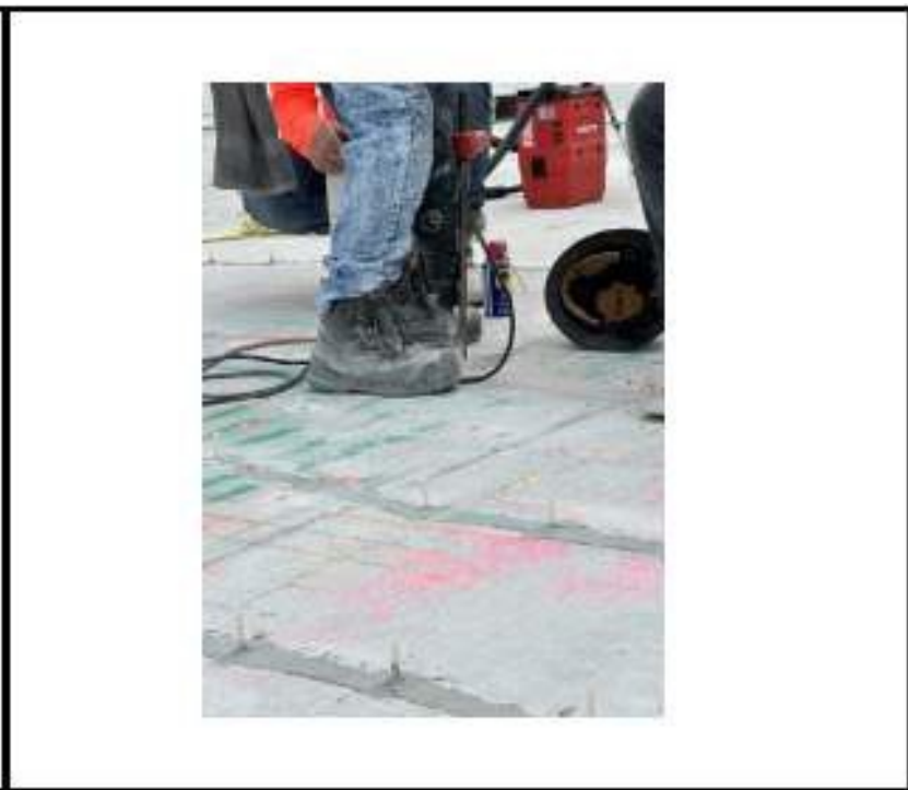
Figure 54. Photograph from Threshold Inspection Report No. 201 showing epoxy crack injection of cracks in roof slab.
