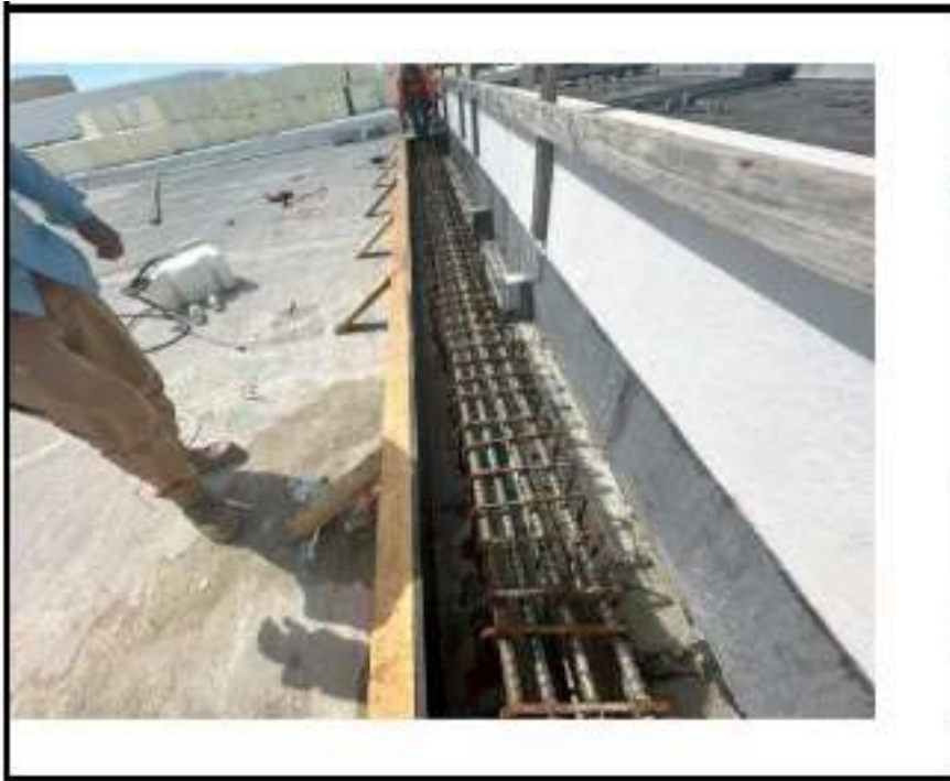
Figure 57. Photograph from Threshold Inspection Report No. 207 showing completed installation of reinforcement in in upturned beam.
