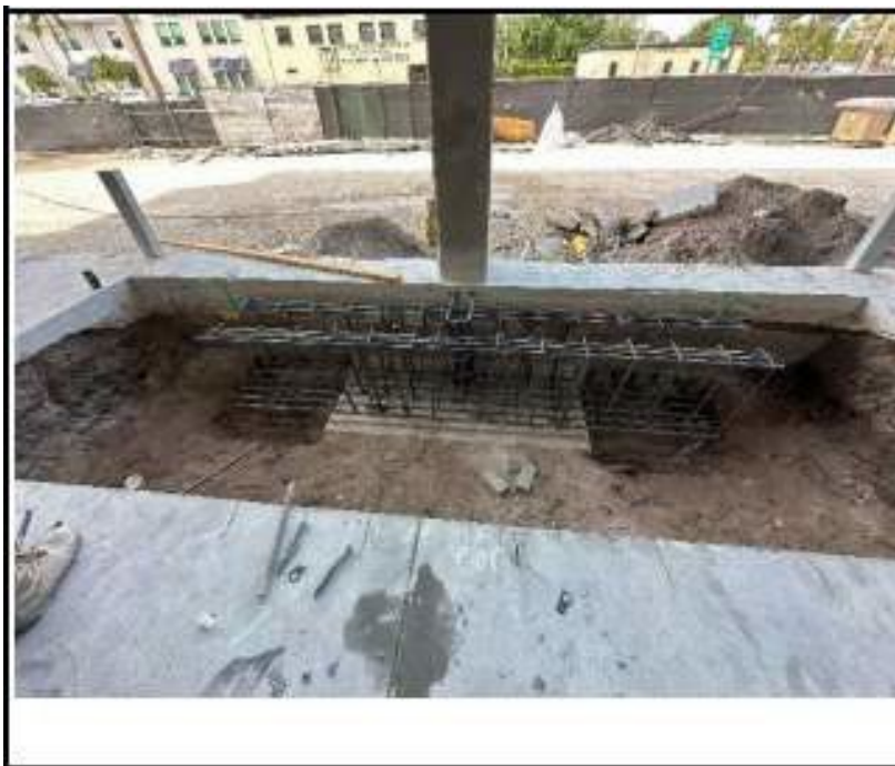
Figure 44. Photograph from Threshold Inspection Report No. 140 showing continuing work on column footing enlargement.
